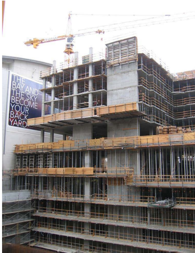
FIGURE 3-3 A shear wall in a concrete structure
