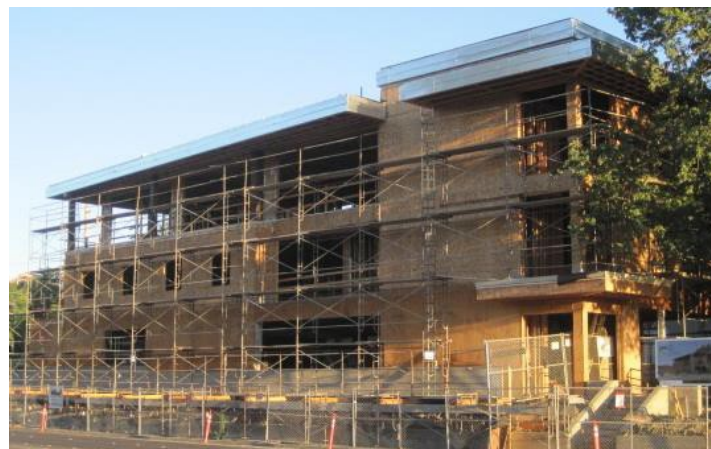
FIGURE 6-3 Commercial wood-frame building
