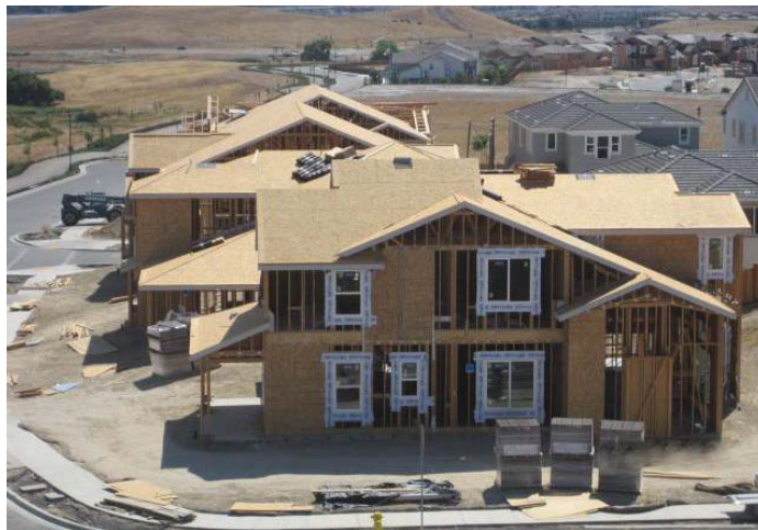
FIGURE 6-1 Single-family residential wood-frame construction
