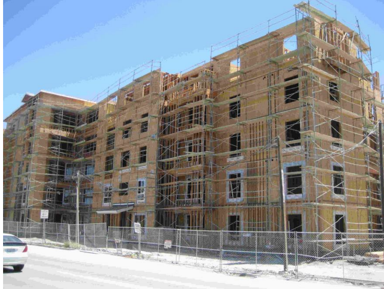
FIGURE 6-2 Multi-family residential wood-frame construction
