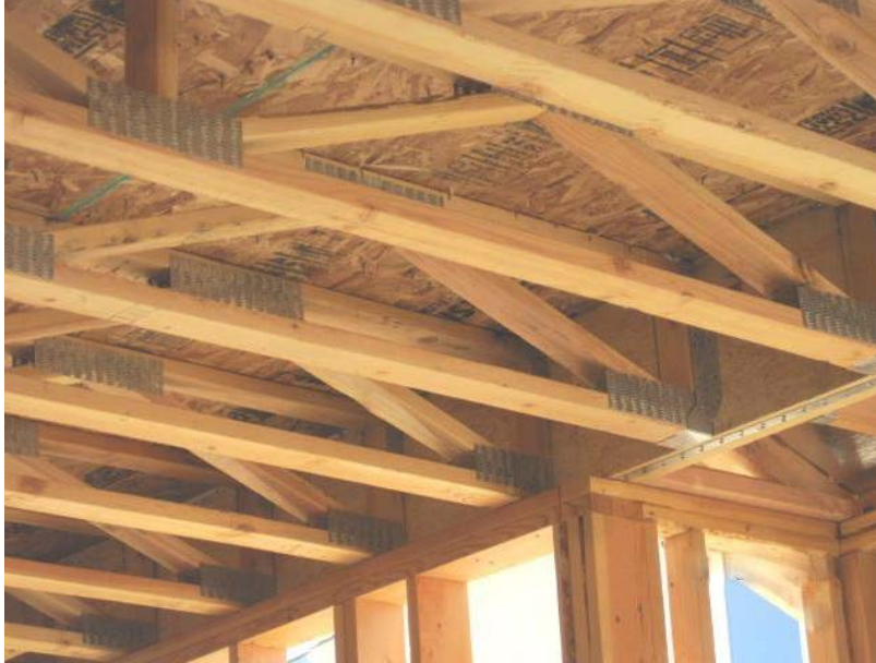
FIGURE 6-6 OSB floor diaphragm on engineered wood trusses
