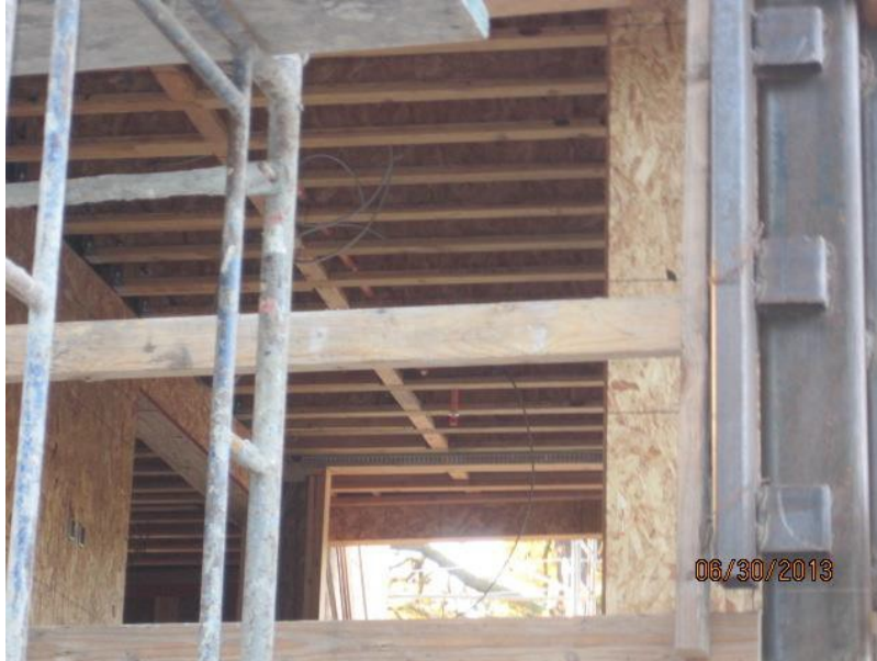
FIGURE 6-5 I-joist framing members
