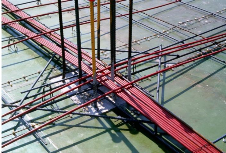
FIGURE 3-2 Post-Tensioned Slab Reinforcement at Column
