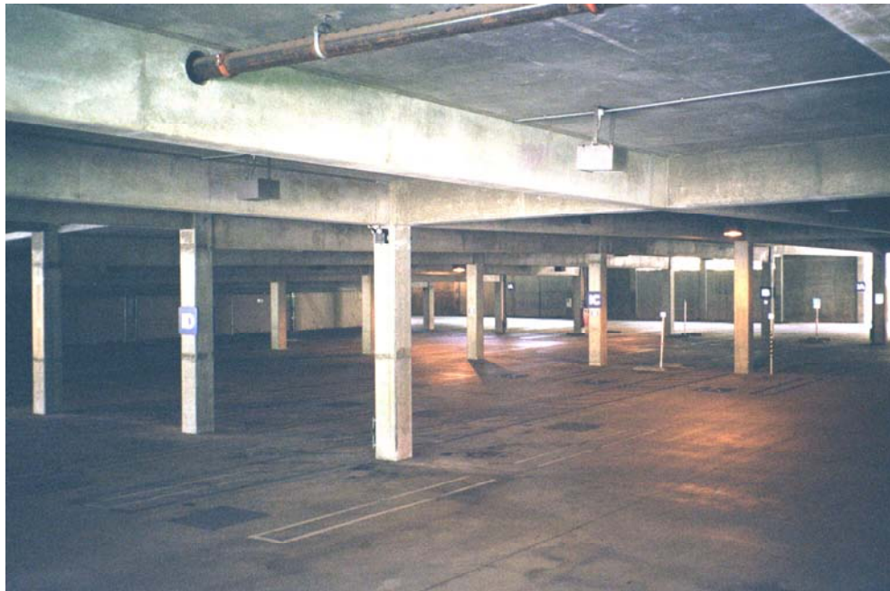
Figure 3-12 Interior view showing concrete columns and girders, which indicate a concrete moment frame (C1).
