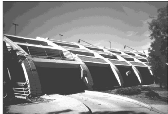
Figure E-26 Extreme example of ductility in concrete, 1994 Northridge earthquake.
