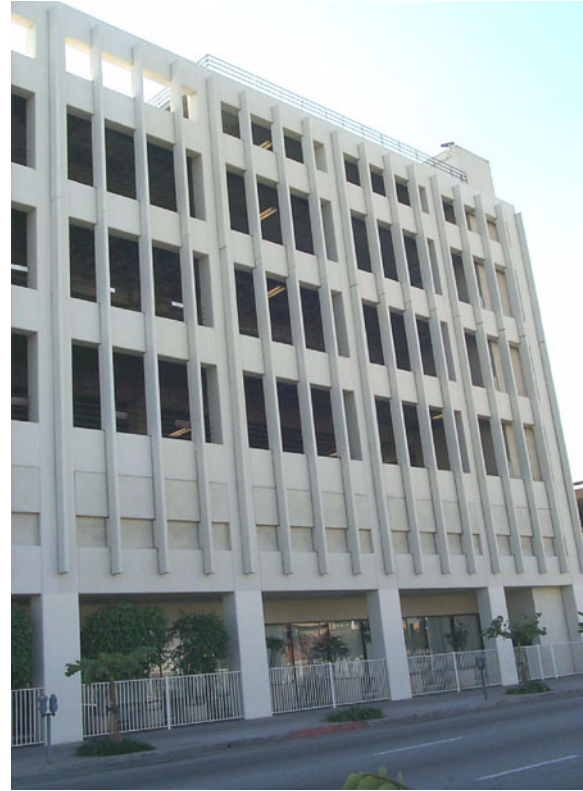
Figure E-28 Concrete moment-resisting frame building (C1) with exposed concrete, deep beams, wide columns (and with architectural window framing).
