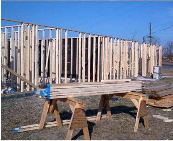
Figure E-4 Stud wall, wood-framed house.
