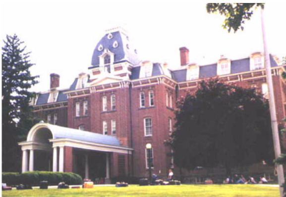
Figure E-50 East coast URM bearing-wall building.
