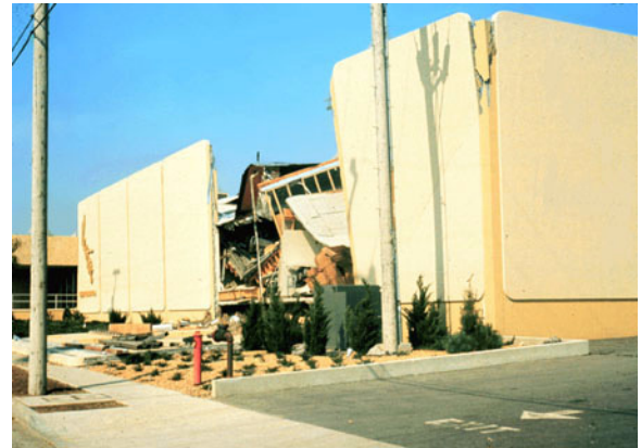
Figure F-12 Collapse of a tilt-up bearing wall.
