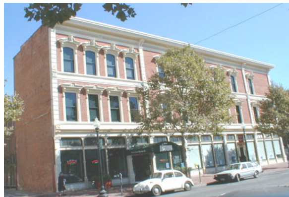
Figure E-51 West coast URM bearing-wall building.
