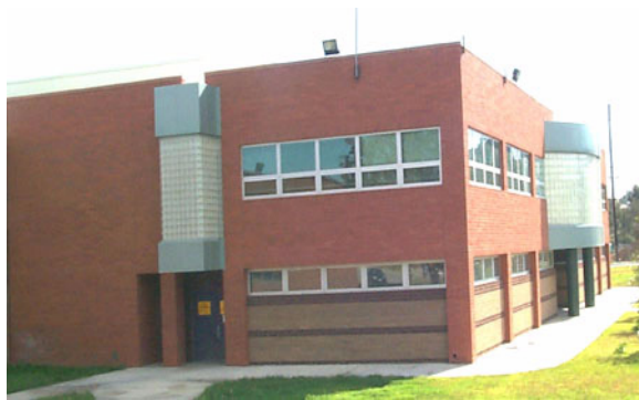
Figure E-46 Modern reinforced brick masonry.
