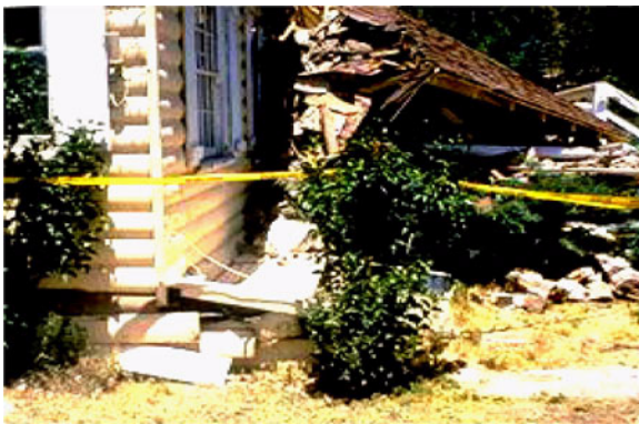
Figure F-9 Collapsed cripple stud walls dropped this house to the ground, 1992 Landers and Big Bear earthquakes.
