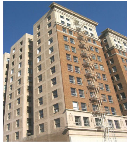
Figure E-33 Concrete frame with URM infill.
