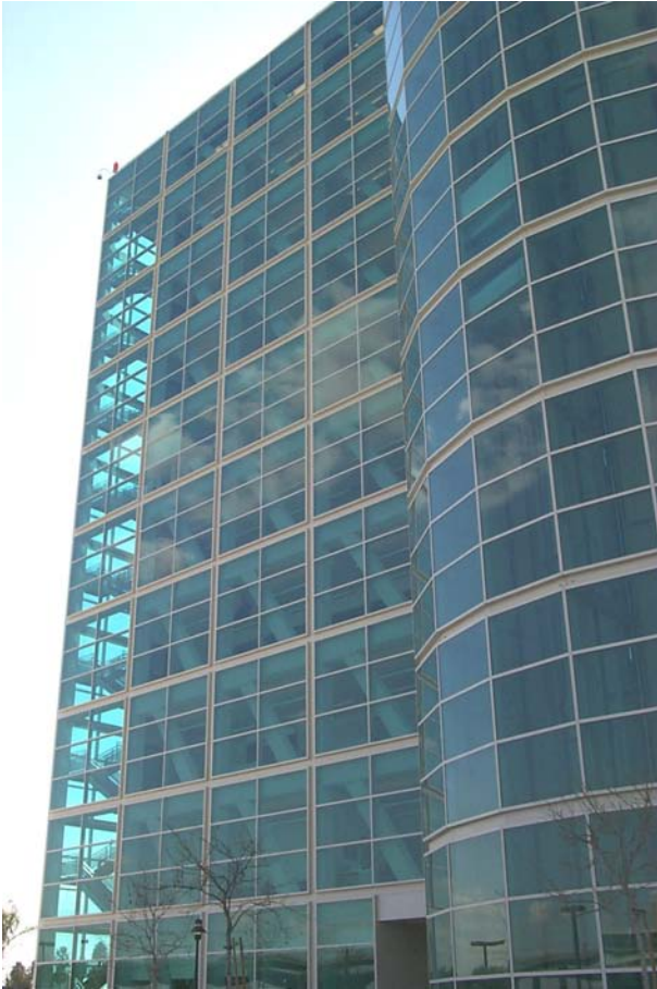
Figure 5-5 Exterior view of 3703 Roxbury Street.
