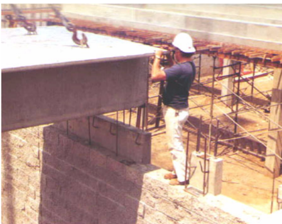
Figure E-44 Example of precast double-T section during installation.
