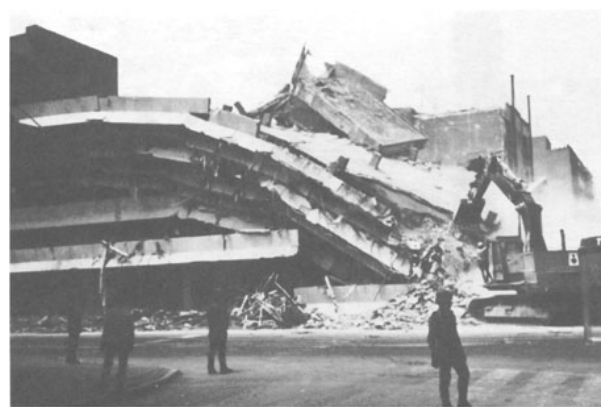
Figure F-5 Mid-rise building collapse, 1985 Mexico City earthquake.
