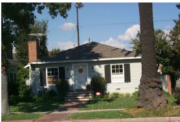
Figure E-1 Single family residence (an example of the W1 identifier, light wood-frame residential and commercial buildings less than 5000 square feet).
