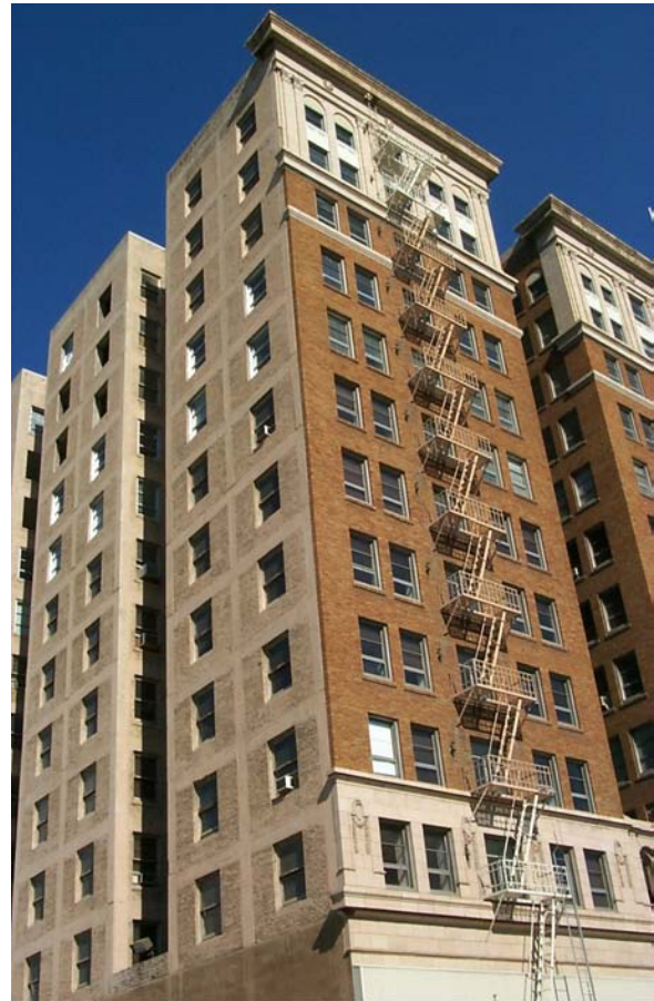
Figure 5-9 Exterior view of 3711 Roxbury.
