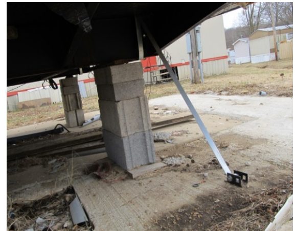
Figure 3-1 Examples of flood and wind tie-down systems for manufactured housing.
