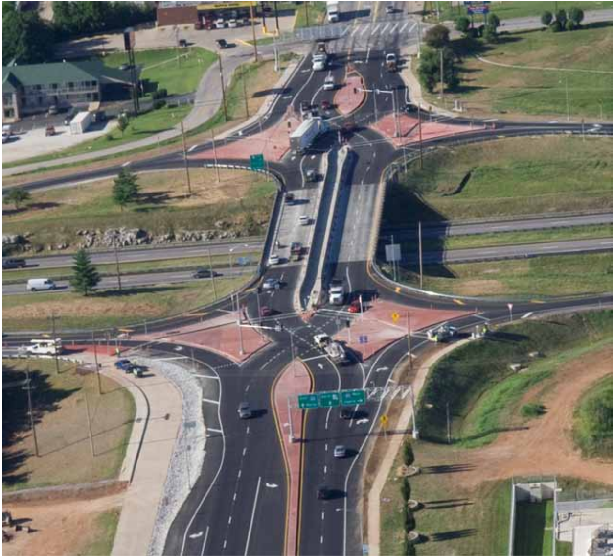
Figure 155. Photo. First U.S. DCD interchange in Springfield, MO.
