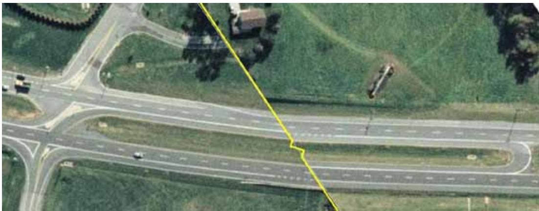
Figure 97. Photo. Auxiliary lanes at J-turn at Emmitsburg, MD.
