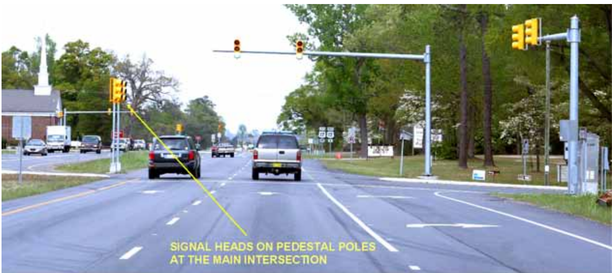
Figure 105. Photo. Signal pole locations at the main intersection of U.S. Route 17 RCUT intersection in North Carolina.
