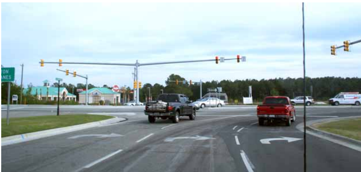
Figure 107. Photo. Signal pole locations at the main intersection from the minor street approach.
