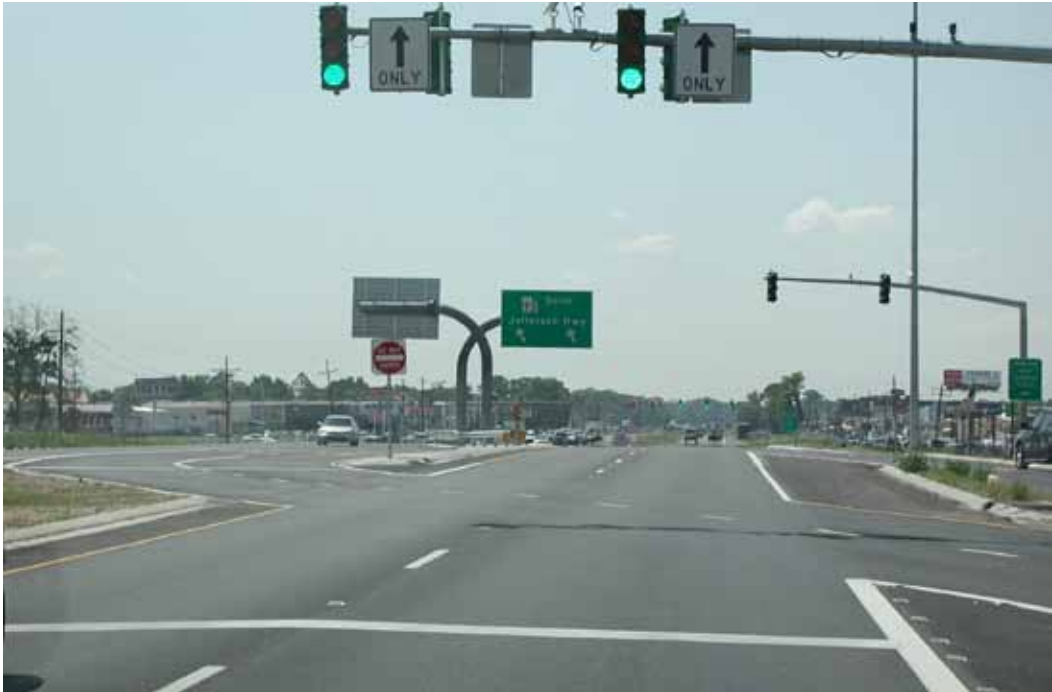
Figure 34. Photo. DLT overhead signing at DLT intersection in Baton Rouge, LA. (11)
