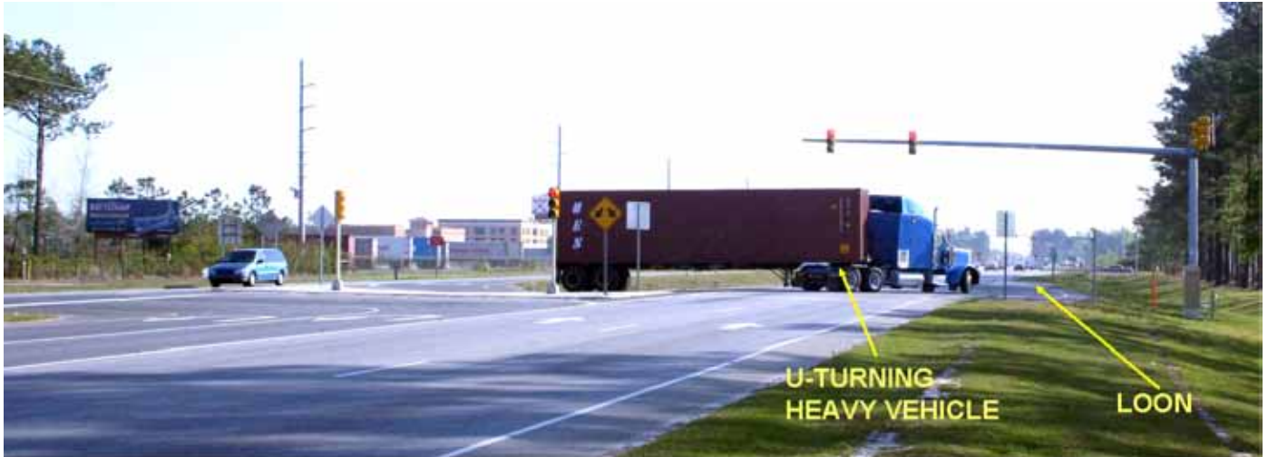
Figure 95. Photo. U-turn movement of a heavy vehicle at a RCUT intersection with a loon on U.S. Route 17 in North Carolina.
