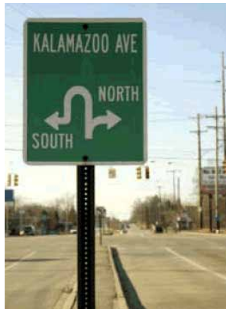
Figure 72. Photo. Example of major road signing used at an MUT intersection in Michigan.
