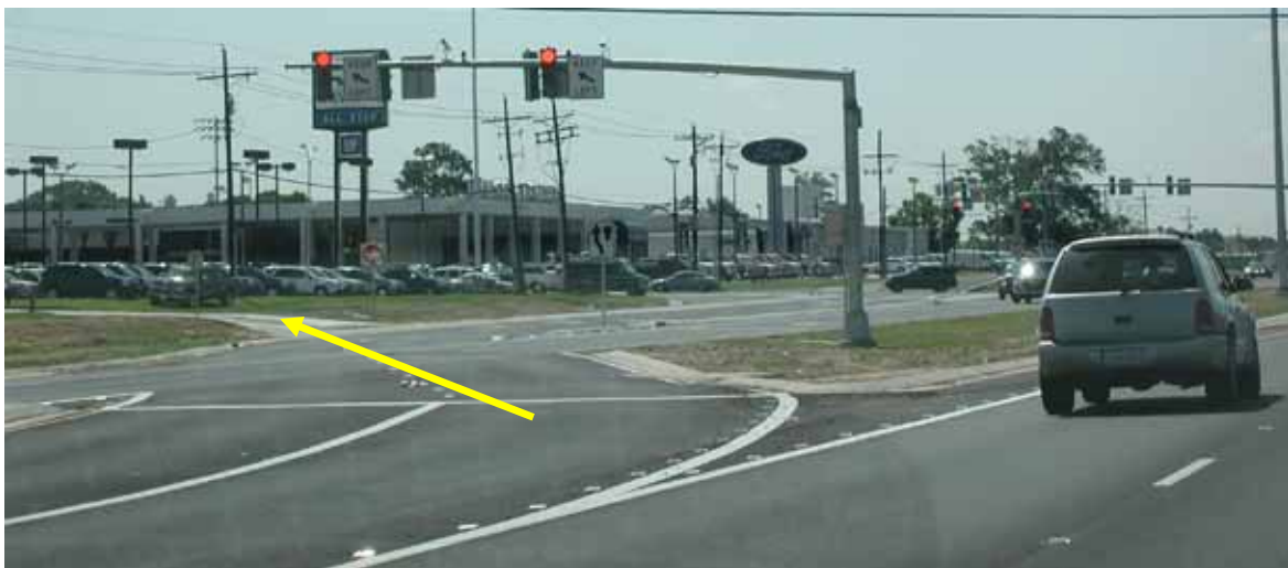
Figure 15. Photo. Right-in, right-out driveway accessible via the right-turn merge lane/frontage road at the DLT intersection in Baton Rouge, LA.
