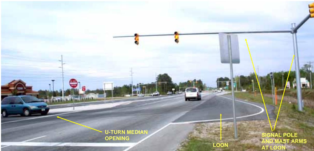
Figure 106. Photo. Signal pole locations at the crossover of U.S. Route 17 RCUT intersection in North Carolina.
