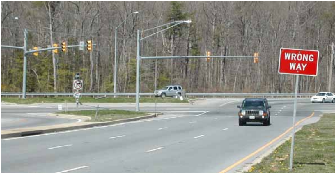
Figure 30. Photo. Signal pole locations at the main intersection viewed from the minor street approach.
