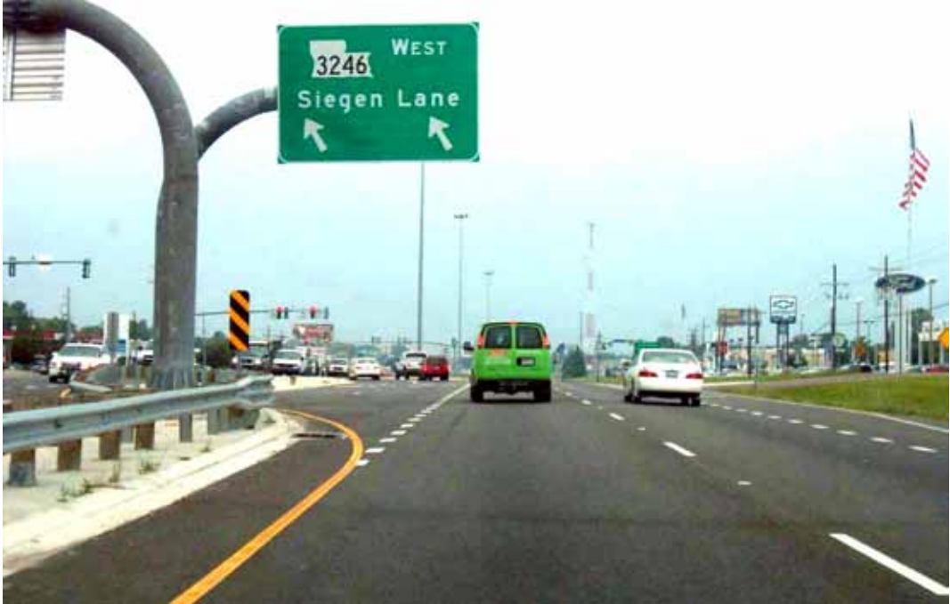
Figure 33. Photo. Overhead signing at the DLT intersection in Baton Rouge, LA. (11)
