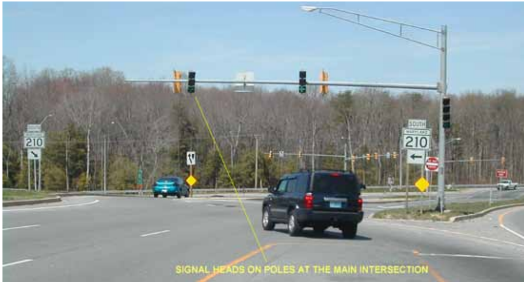
Figure 27. Photo. Signal pole locations at the cross junction at the intersection of MD 210 at MD 228 in Accokeek, MD.
