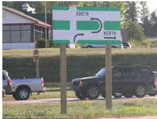
Figure 71. Photo. Example of alternative minor road signing used at an MUT intersection in Michigan.
