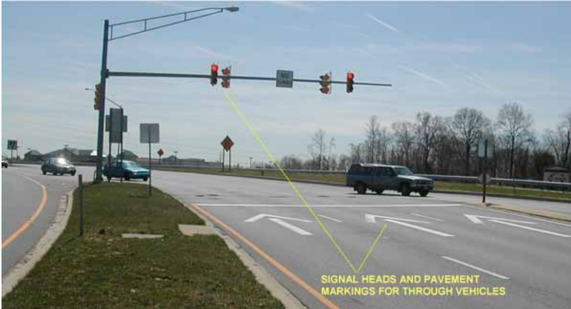
Figure 29. Photo. Signal pole locations at the intersection of MD 210 at MD 228 in Accokeek, MD.
