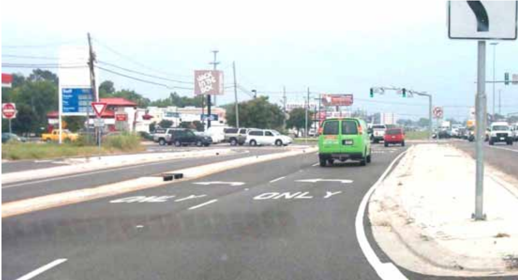
Figure 35. Photo. Pavement markings on the displaced left-turn lanes at DLT intersection in Baton Rouge, LA. (11)
