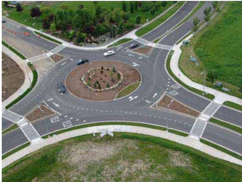
Figure 142. Photo. Typical roundabout.
