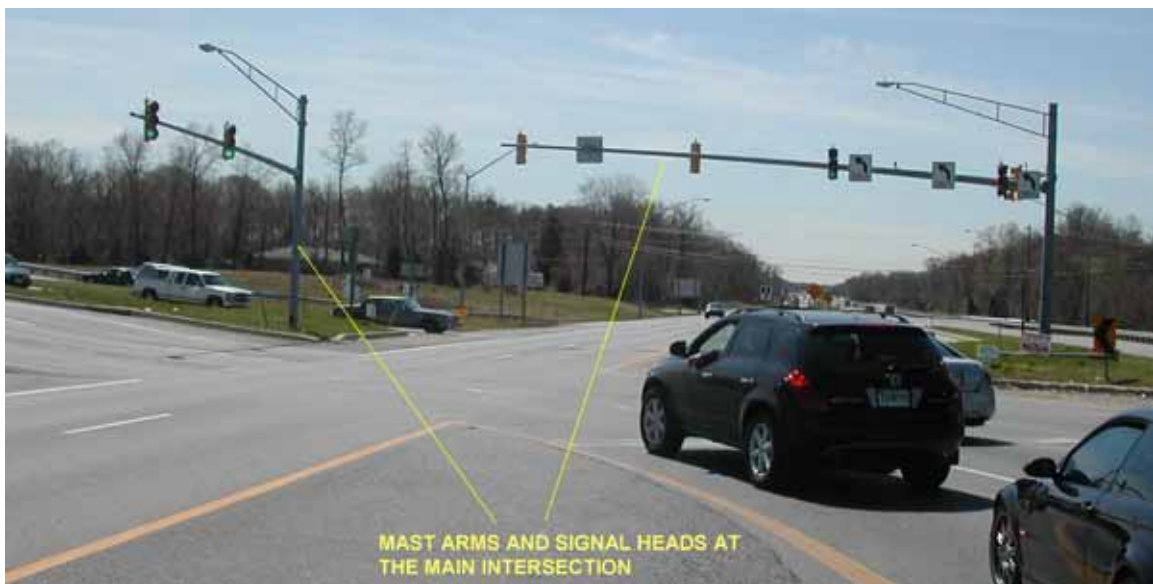
Figure 28. Photo. Signal pole locations at the main intersection of MD 210 at MD 228 in Accokeek, MD.
