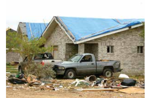
PHOTO: FEMA-provided "blue tarp" temporary roof protection.
