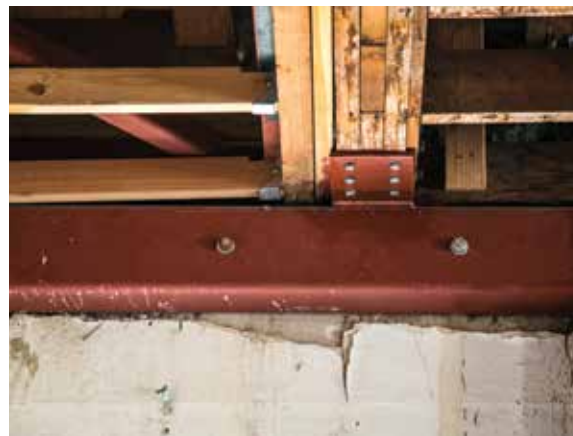
PHOTO: Steel structural support added for earthquake resistance.
