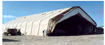
Large Area Maintenance Shelter (Clamshell) (Army/Navy/Air Force)
