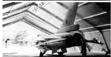
TOP: BEAR Program - Dome Shelter (Air Force), BOTTOM: Interior View Aircraft Hangar
