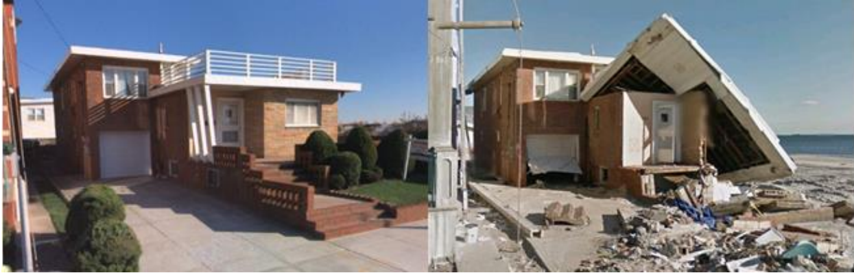
Figure 8. Wave and Erosion Damage, Rockaway Beach, NY.
