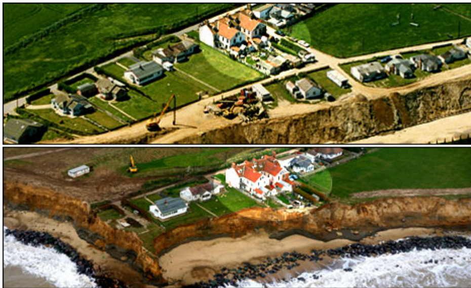
Figure 8.3: Progressive coastal erosion of bluffs at Happisburgh, village, east coast of United Kingdom comparing situation in 1981 (top) with 2008 (bottom)
