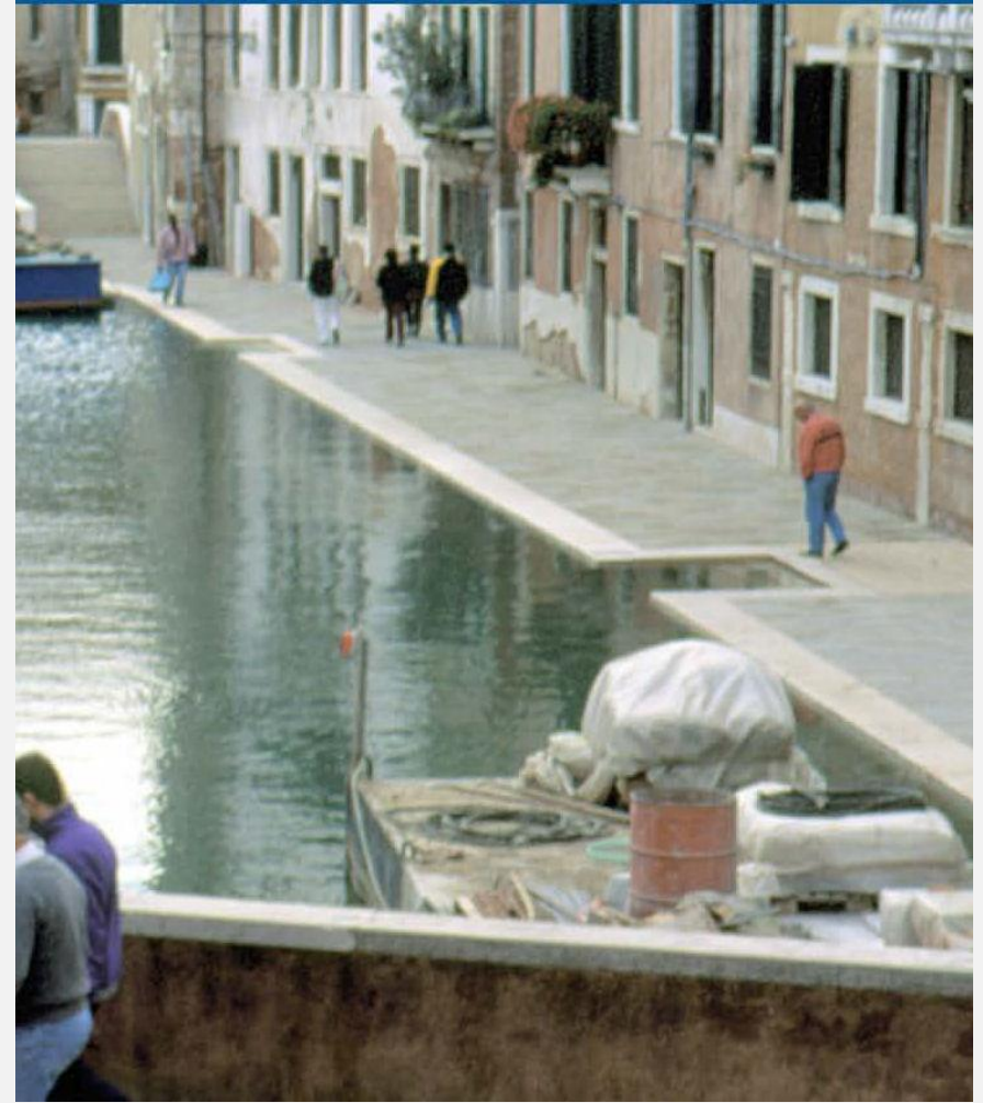
After Raising of banks and pavements
