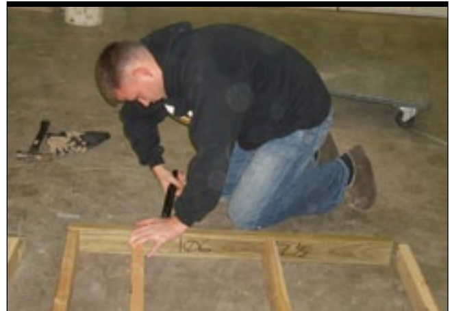
Marine Corps Sgt. Adam Walker constructs wall framing.
