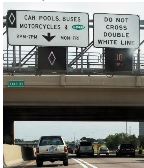
Figure 4. Photo. Example of a tolled high-occupancy vehicle lane separated by lane markings from normal travel lanes.
