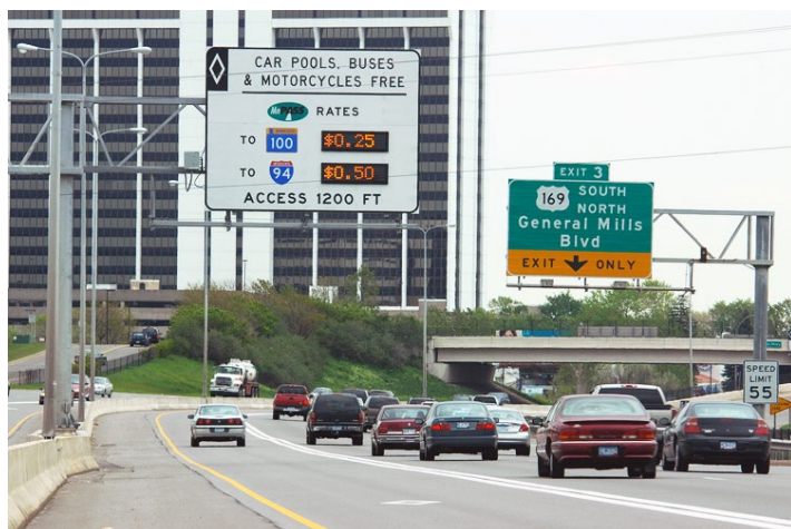
Figure 12. Photo. A sign on a gantry shows rates for using a high-occupancy toll lane to reach different destinations.
