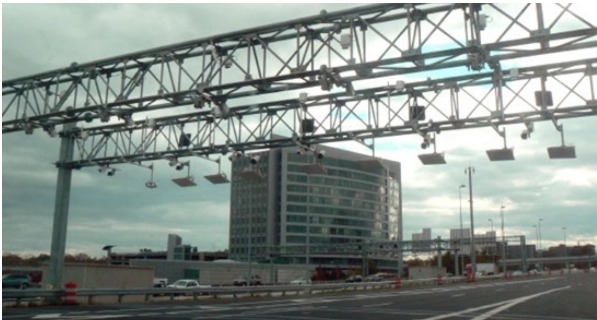
Figure 14. Photo. Video and transponder detection devices mounted on an overhead gantry on the I-495 Express Lanes in Virginia.
