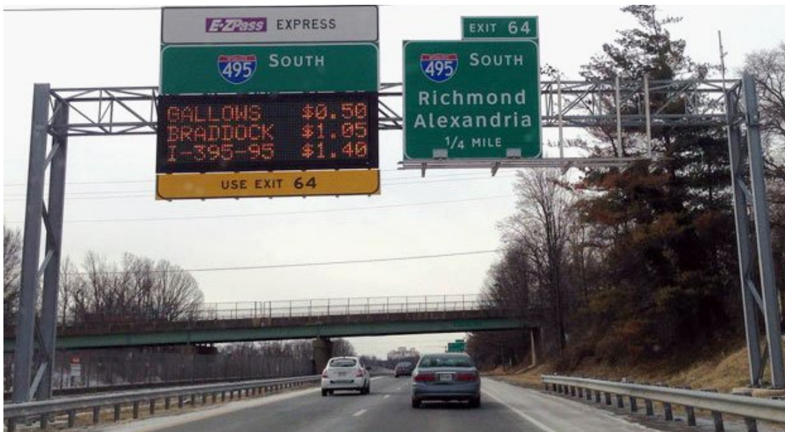
Figure 15. Photo. A dynamic sign mounted on a gantry depicts the cost to travel to different destinations using the I-495 Express Lanes.
