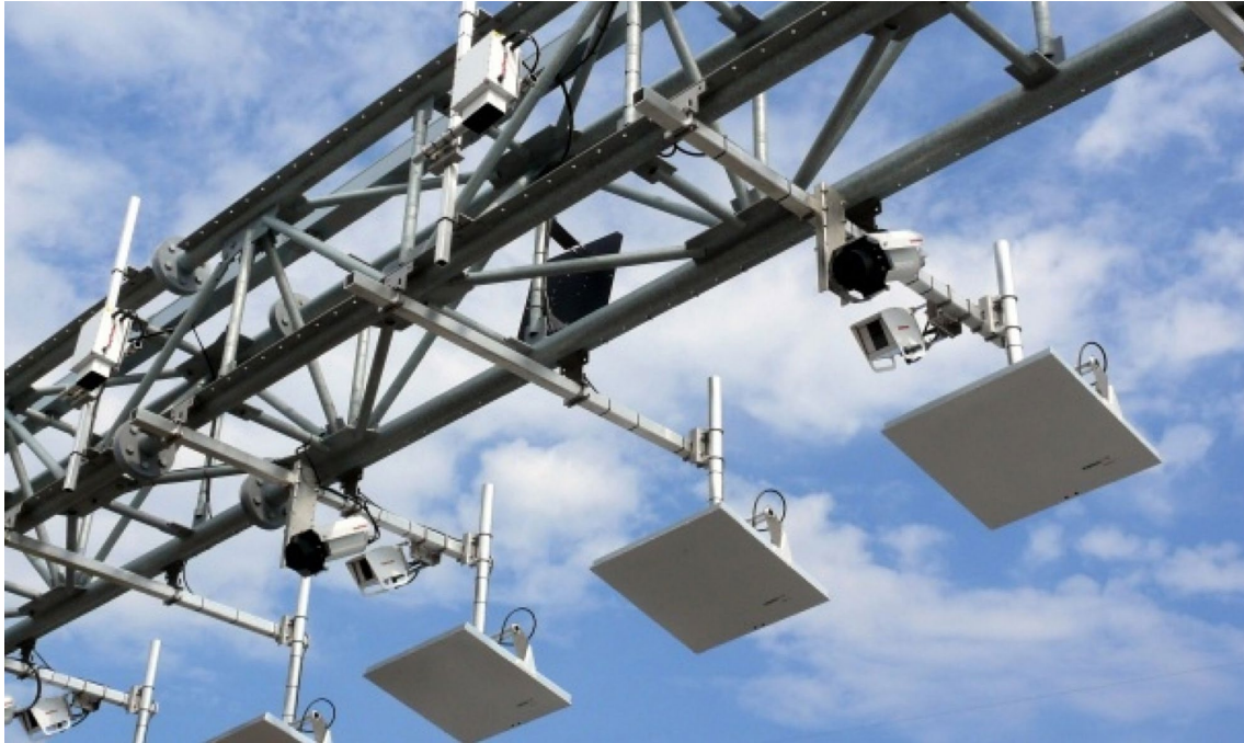
Figure 7. Photo. Video and transponder detection devices mounted on an overhead gantry.
