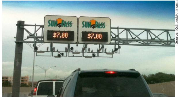
Figure 6. Photo. Changeable displays on an overhead gantry indicate the cost of using SunPass tolled lanes in Florida.
