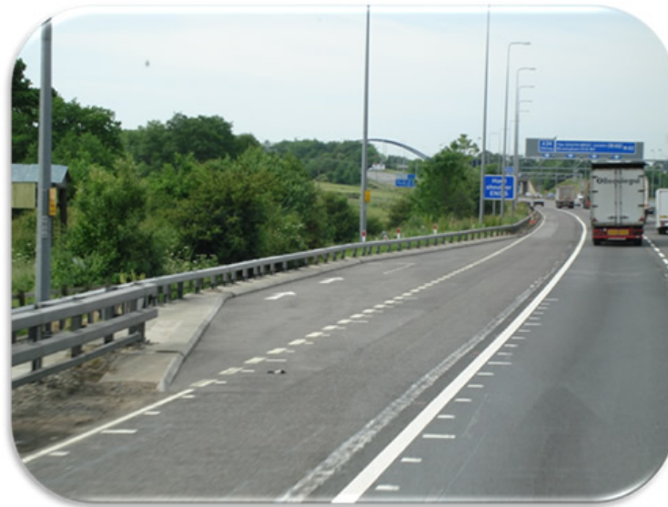
FIGURE 19. PHOTOGRAPH. EMERGENCY REFUGE AREA IN THE UNITED KINGDOM (13)
