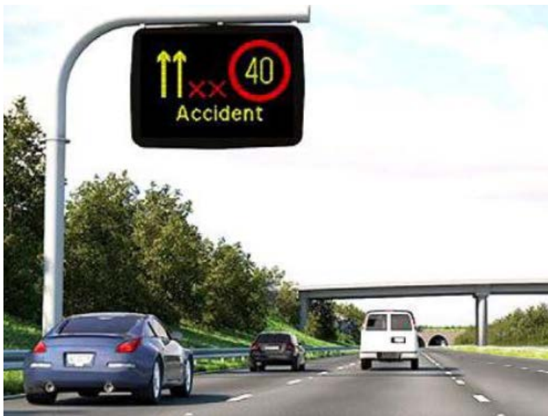
FIGURE 26. PHOTOGRAPH. CONCEPTUAL VERGE (SIDE)-MOUNTED SIGN FOR ACTIVE TRAFFIC MANAGEMENT (ATM) AS STUDIED IN THE UNITED KINGDOM (46) (Source: UK Highways Agency)
