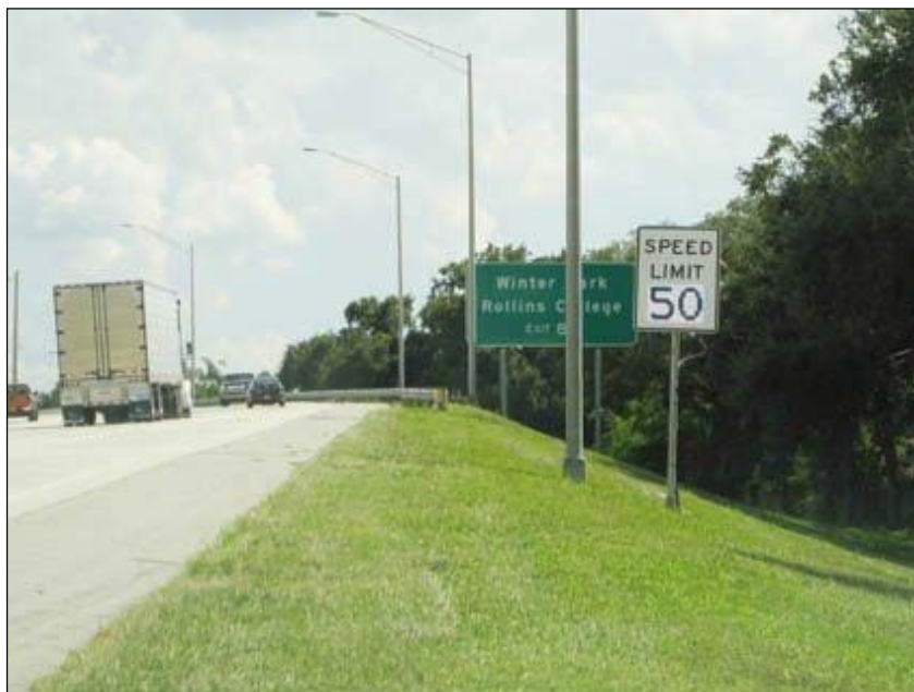
FIGURE 15. PHOTOGRAPH. EXAMPLE OF SIDE-MOUNTED DYNAMIC SPEED LIMIT (DSPL) SIGN (Source: Florida DOT)
