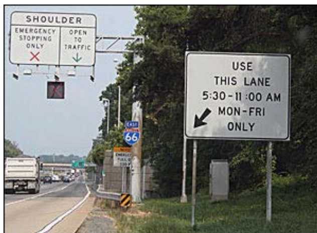
FIGURE 28. PHOTOGRAPH. DYNAMIC SHOULDER LANE (DShL) SIGNAGE IN NORTHERN VIRGINIA (Source: Virginia DOT)
