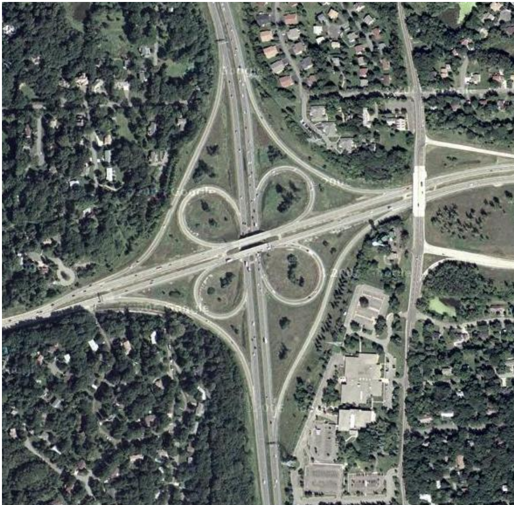
Figure 2: Intersection of Interstate 494 and TH 7 in Minneapolis, Minnesota
