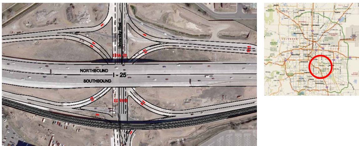
Figure 10: I-25 Interchange in Denver, Colorado
