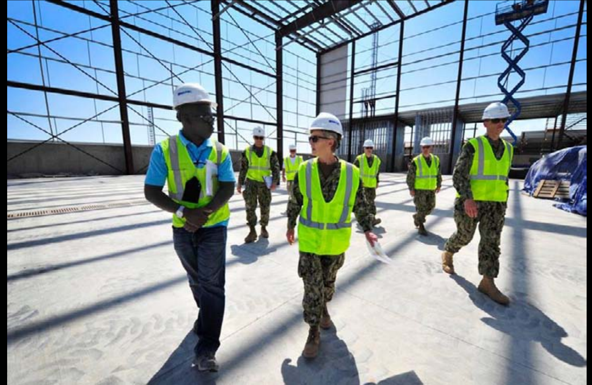
Chief of Civil Engineers, Rear Adm. Katherine Gregory, center, discusses a building construction development plans with Eric Ofei, a Camp Lemonnier construction site manager. Gregory and Seabee Force Master Chief Christopher Levesque are conducting site visits throughout the European Region to assess various engineering support facilities and bases. (U.S. Navy photo by Mass Communication Specialist 1st Class Julia A. Casper/Released)
