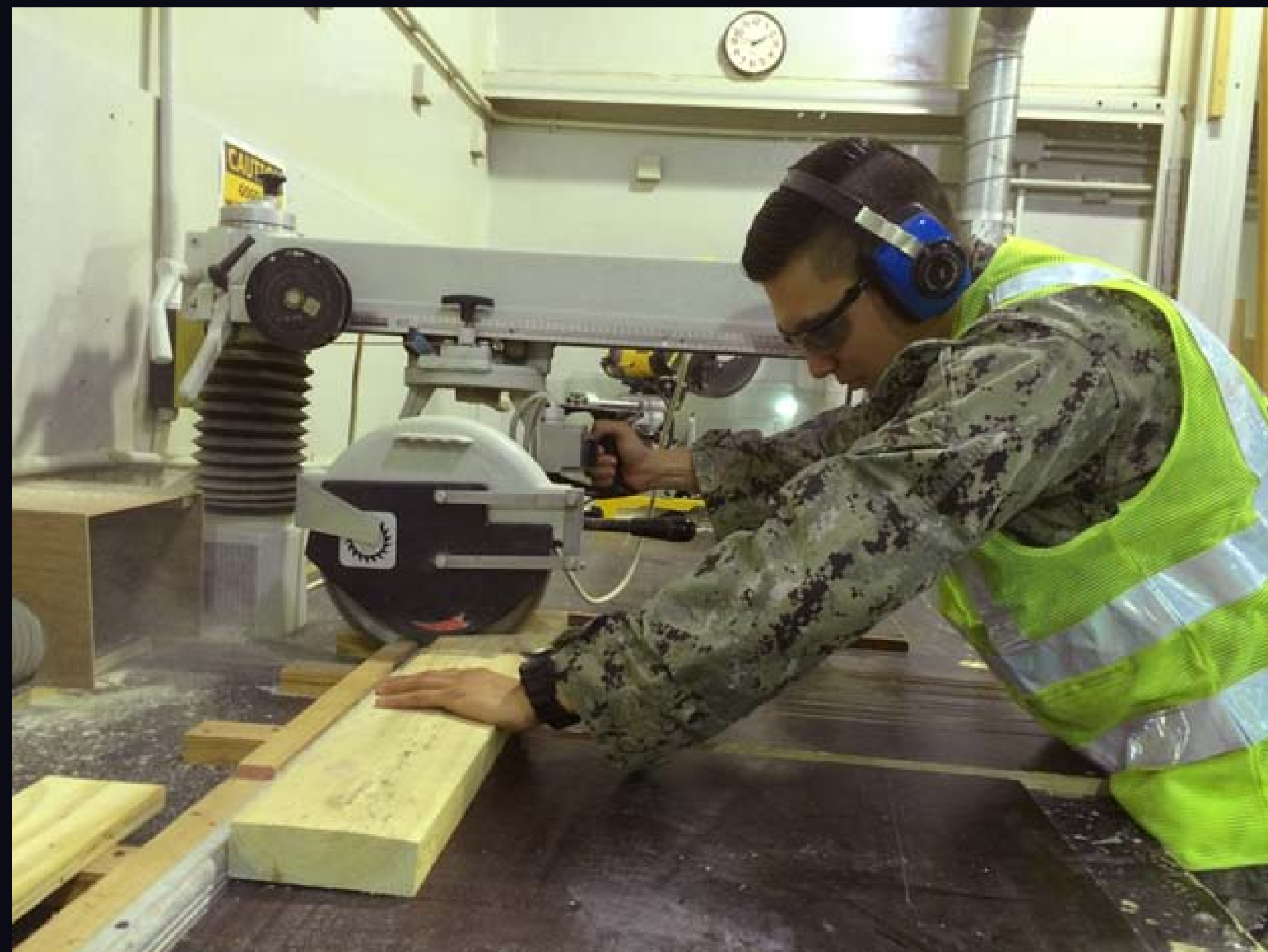
Builder Third Class (BU3) Juan Orosco cuts a 2x6 at the Public Works Department (PWD) Bahrain Builder Shop. The lumber will be used in a project to replace a damaged staircase and railing, currently posing a safety hazard, for Morale Welfare and Recreation (MWR) Fitness Center onboard Naval Support Activity (NSA) Bahrain. (U.S. Navy photo by PWD Bahrain)
