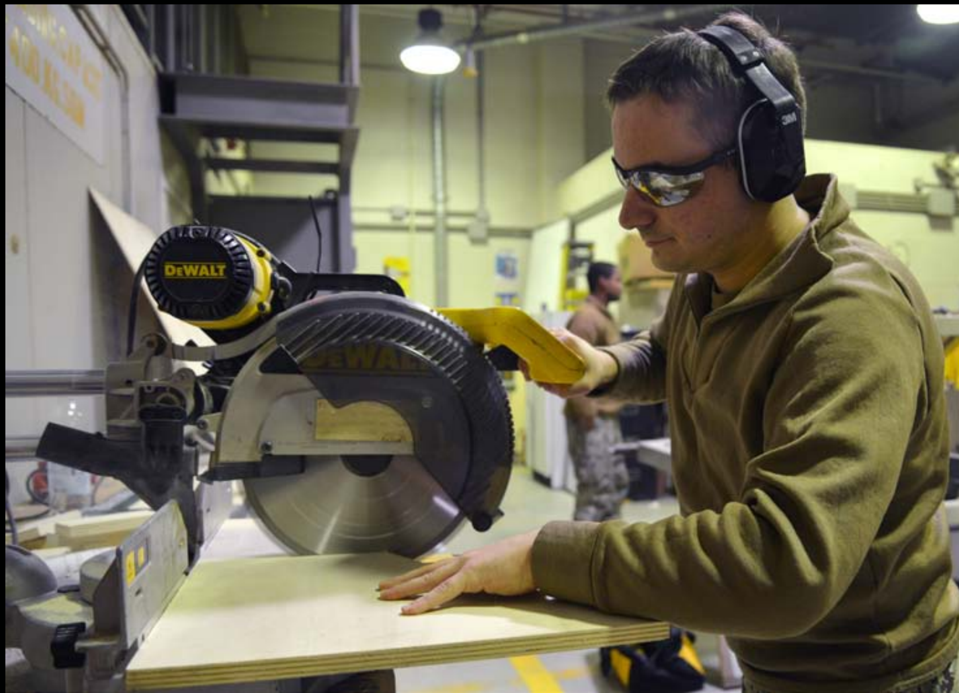
Builder 2nd Class Eric Kraninger, assigned to Public Works Department Naples, Italy uses a Miter saw to cut pieces of wood in the production shop Jan. 28, 2015. PWD Naples provides a full range of NAVFAC construction, engineering, facility maintenance, utilities, transportation and environmental services to NSA Naples and tenant commands. (U.S. Navy photo by Mass Communication Specialist 2nd Class Eva-Marie Ramsaran/Released)
