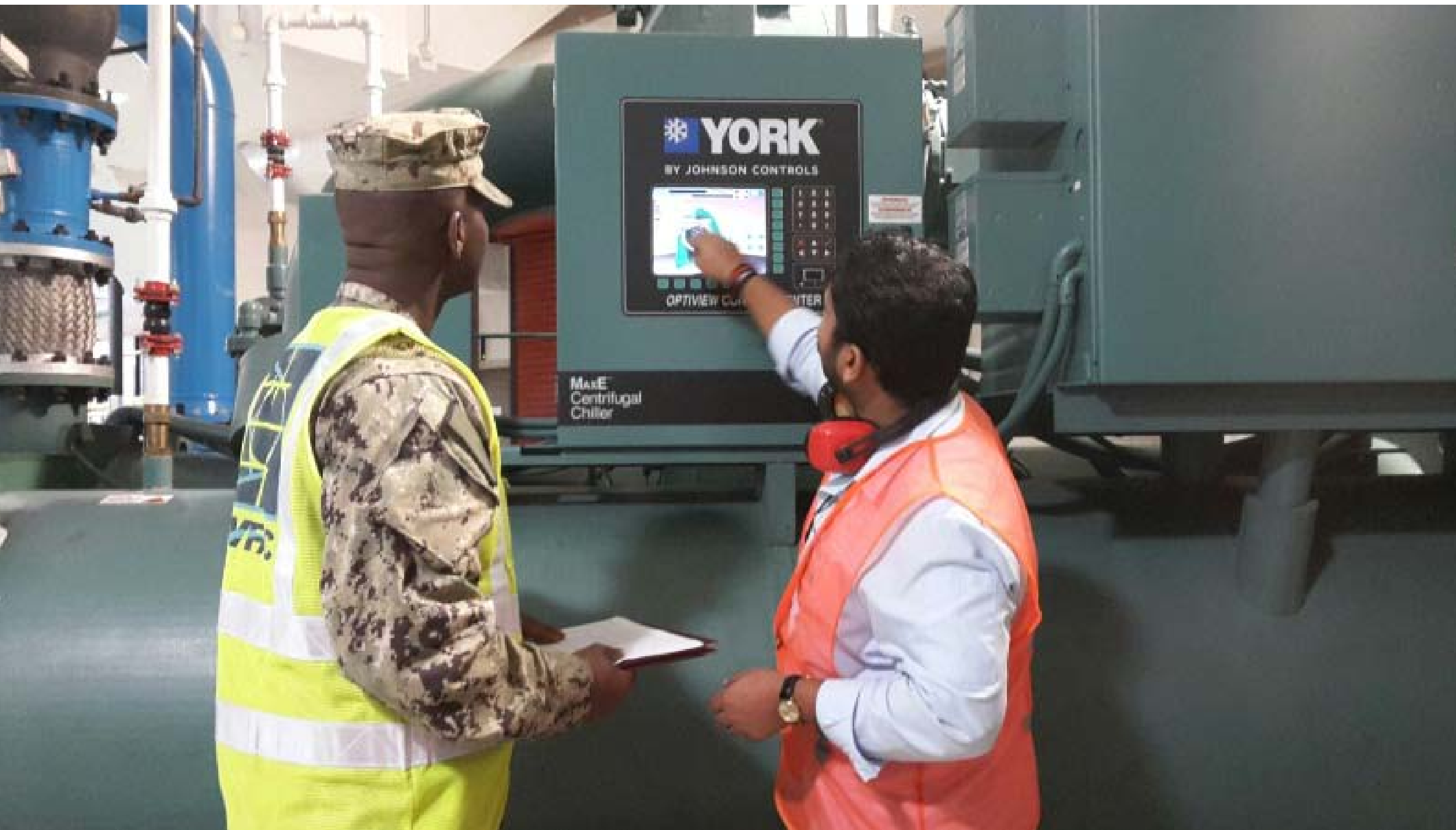
EA1 Barezi verifies the centrifugal chiller log sheet data during an unscheduled performance assessment inside the Combined Utility Building (CUB). The chillers keep NSA 2 facilities at pleasant temperatures, even during the brutal Bahraini summers when the mercury often pushes 110 degrees. (U.S. Navy photo by NSA Bahrain/Released)
