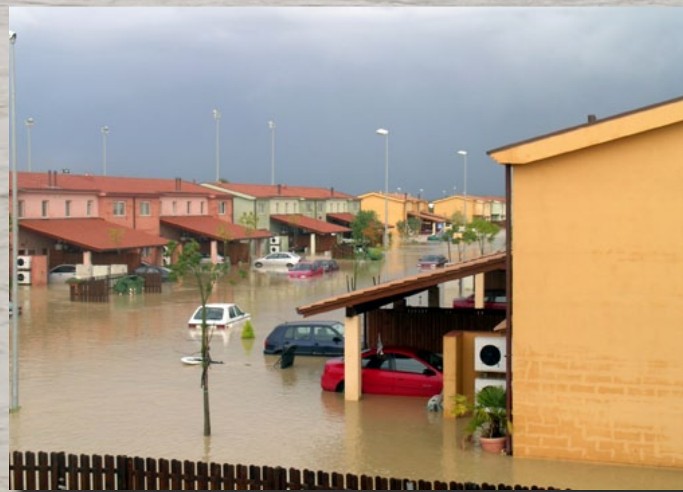
U.S. Navy family housing complex in the town of Maranai. Continuous heavy rainfall resulted in flooding and power outages aboard Naval Air Station (NAS) Sigonella and in surrounding areas, including government housing units in the towns of Maranai and Maneo. Six inches to three feet of standing water was reported. NAS Sigonella provides logistical support to Commander 6th Fleet in support of the Global War on Terrorism. U.S. Navy photo by Utilitiesman Chief Jody Markham (RELEASED)
