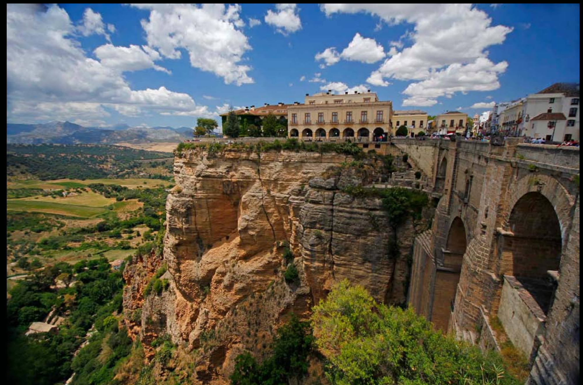
The view of the Puente Nuevo, or New Bridge in English, in the town of Ronda, located in the picturesque Andalusia mountains of Spain. (U.S. Navy Photo by Chief Mass Communication Specialist William Clark/Released)
