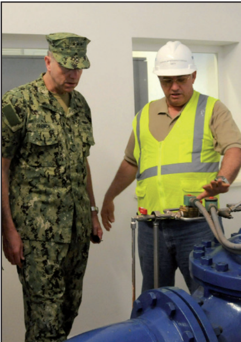
Commander, Navy Installations Command Vice Adm. William D. French receives a brief from Rota's Public Works Department General Maintenance Foreman Larry Smith at the installation's water treatment facility. (Photo by MC2 Travis Alston/Released)
