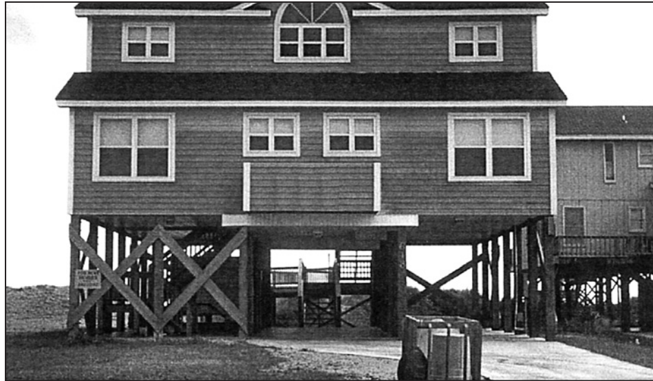
Figure 10-10. Diagonal bracing using dimensional lumber
