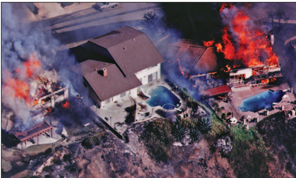
Figure 11-3. House that survived a wildfire due in part to fire-resistant walls and roof while surrounding houses were destroyed SOURCE: DECRA ROOFING SYSTEMS, USED WITH PERMISSION
