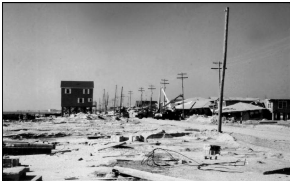
Figure 11. Hurricane Hugo (1989), Garden City Beach, SC. House on pilings survived while others did not.
