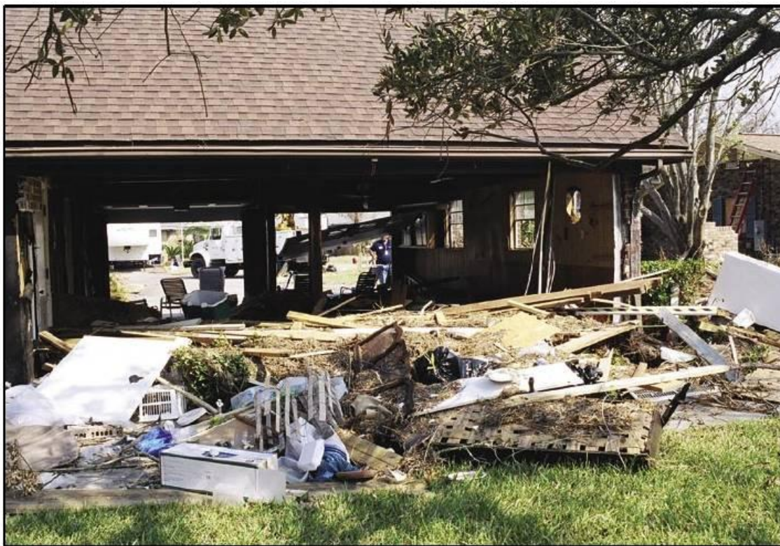
Figure 20. This house, located in Zone AE, experienced Zone V surge and wave conditions (Santa Rosa Sound, FL, 2004).
