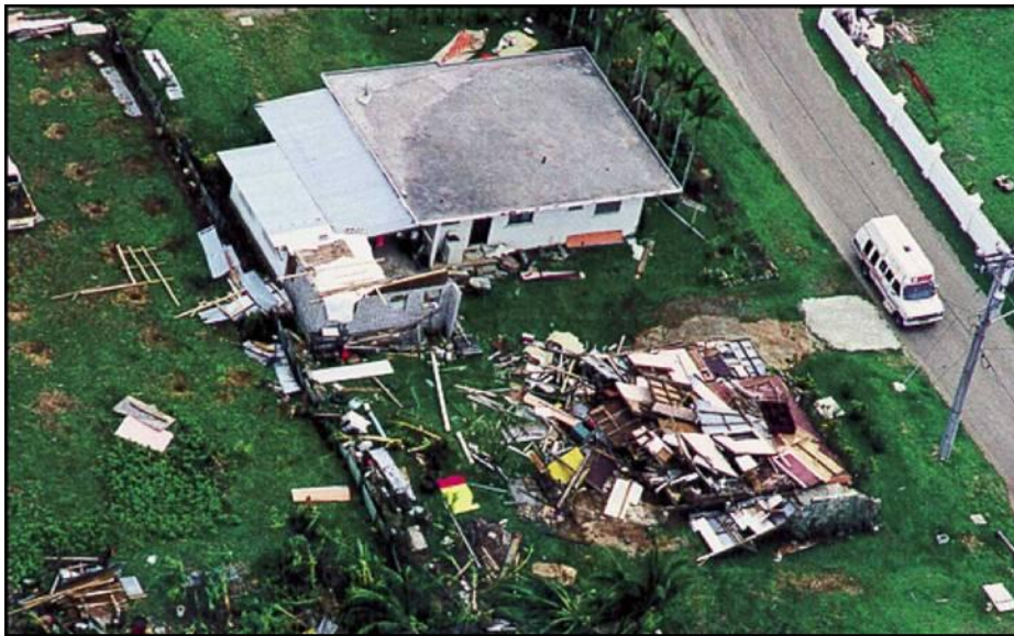
Figure 31. Typhoon Paka (1997). Although damaged by the storm, the concrete house in the upper part of the photograph survived, while the wood-frame house next to it was destroyed.
