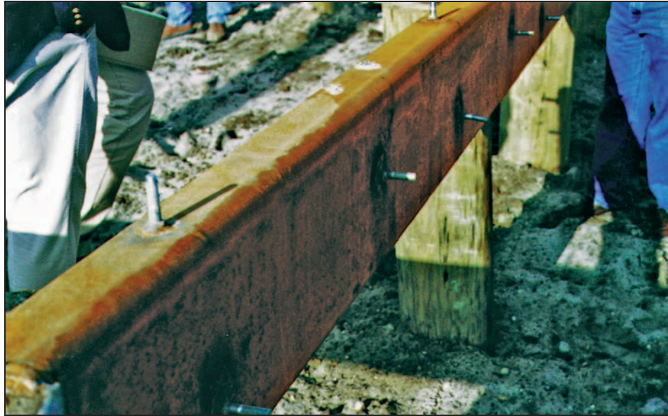
Figure 9-31. House being constructed with a steel frame on wood piles
