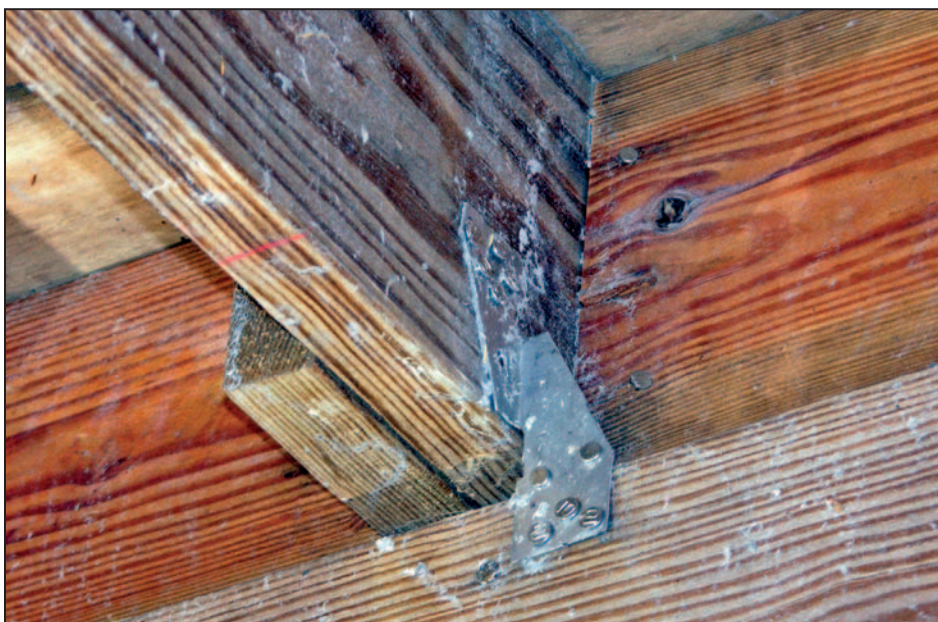
Figure 9-17. Metal joist-to-beam connector
