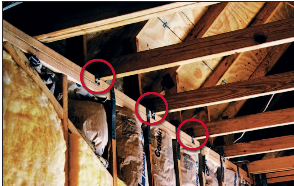
Figure 9-9. Connection of truss to wood-frame wall
