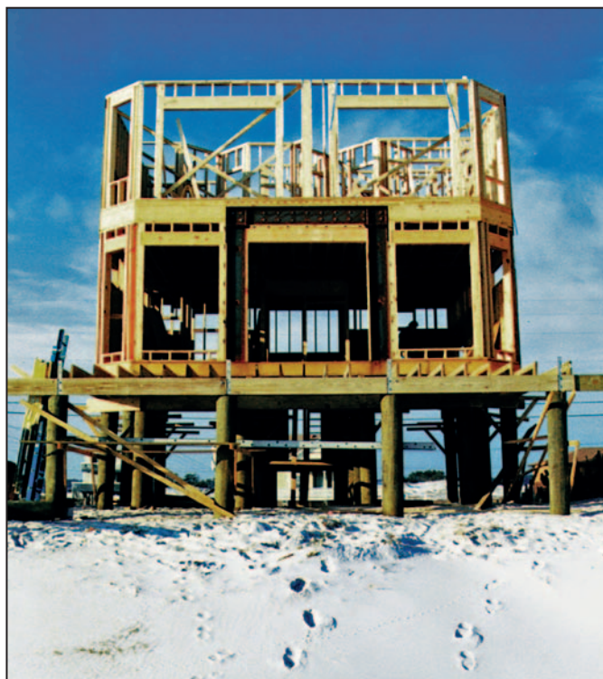
Figure 9-25. Steel moment frame with large opening
