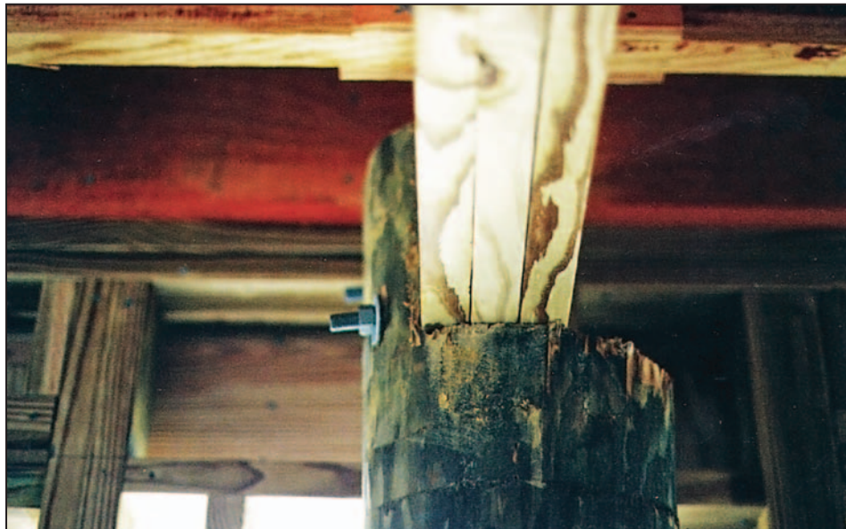
Figure 13-3. Improper overnotched wood pile
