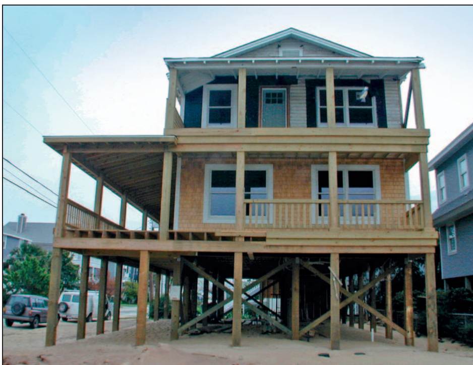
Figure 15-9. Home elevated on piles
