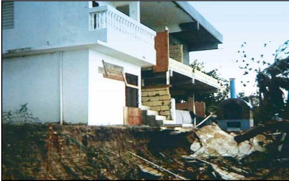
Figure 24. Hurricane Georges (1998). Coastal building in Puerto Rico damaged by storm surge and waves.
