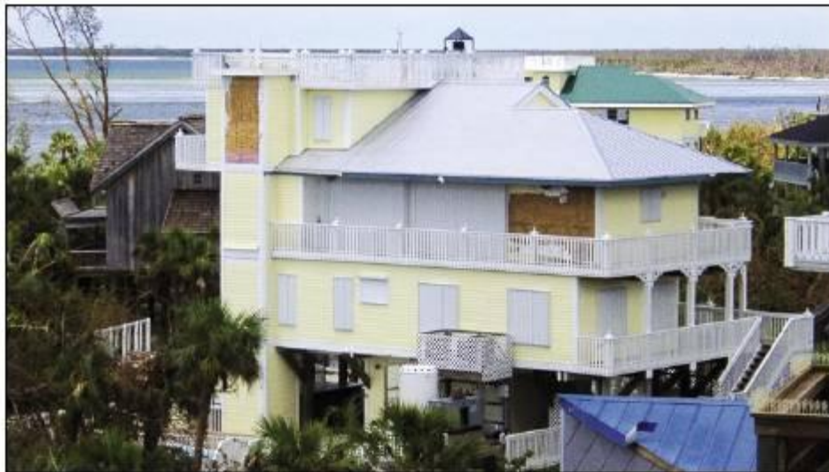
Figure 15. No structural damage was observed to homes built to the 2001 FBC (North Captiva Island, FL, 2004).
