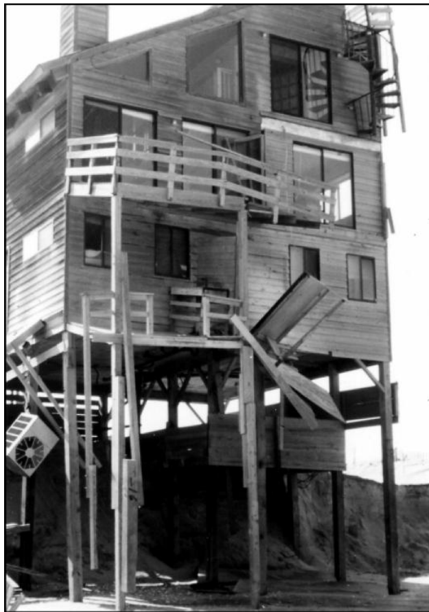
Figure 6. March 1989 nor'easter. Although this house seems only to have lost decks and a porch, the loss of supporting soil compromises its structural integrity.
