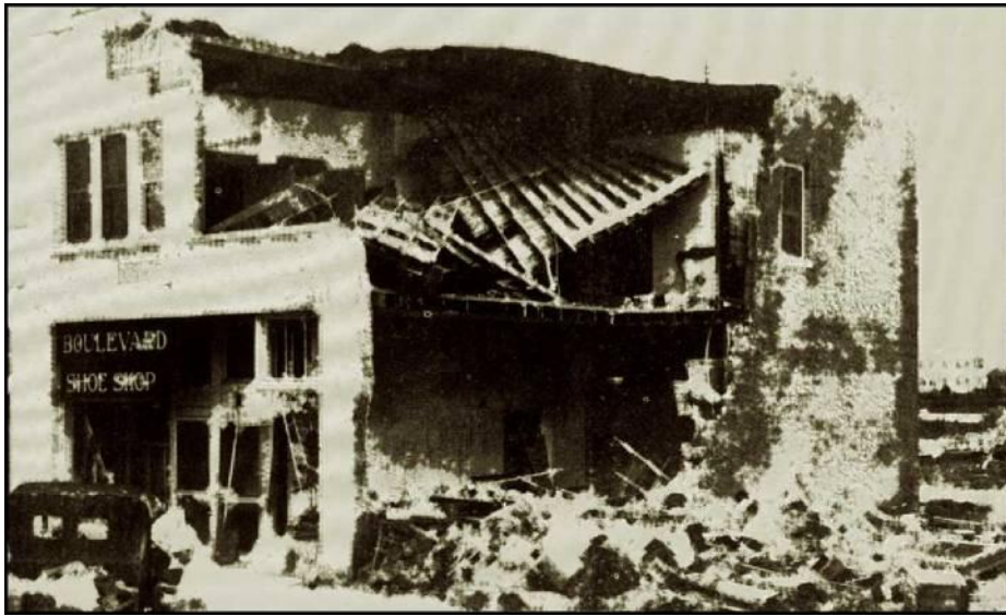
Figure 10. Building damage from 1926 hurricane, Miami, FL.
