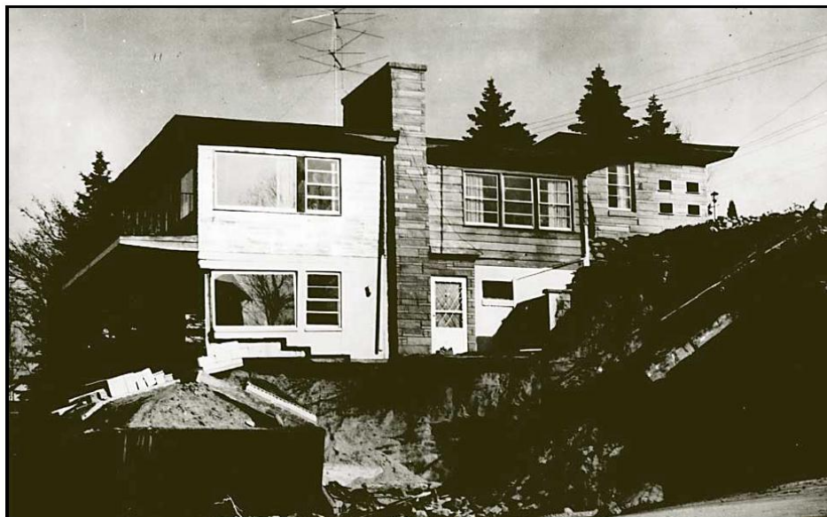
Figure 25. House on southeastern shoreline of Lake Michigan undermined by erosion during storm of November 1951.
