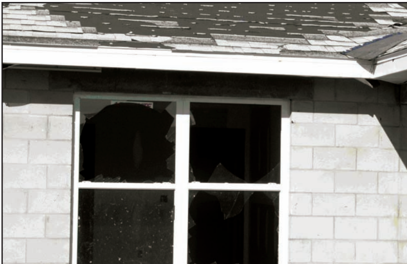
Figure 10-3. PUNTA GORDA, FLORIDA: Glazing failure due to windborne debris from displaced roofing. (Source: FEMA 488)
