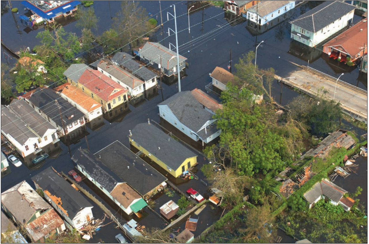
Figure 2-27. NEW ORLEANS, LOUISIANA: Neighborhood with homes flooded and cars covered. In the background is a breached levee with water entering the area. (Source: FEMA 549)
