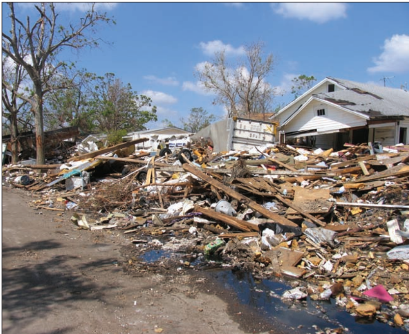
Figure 2-9. GULFPORT, MISSISSIPPI: Floodborne debris, including shipping containers and sections of destroyed buildings. (Source: FEMA 549)
