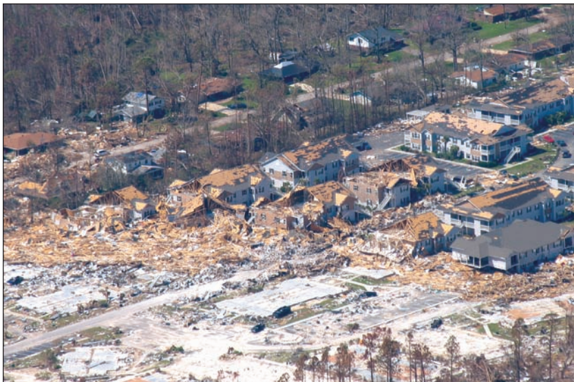
Figure 2-2. LONG BEACH, MISSISSIPPI: Aerial photo of apartment complex and surrounding area after Hurricane Katrina. (Source: FEMA 549)
