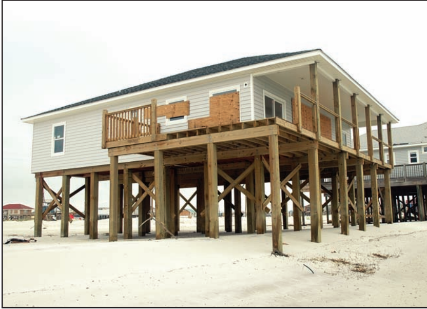
Figure 6-10. DAUPHIN ISLAND, ALABAMA: Successful pile foundation following Hurricane Katrina. The foundation supported the elevated home even after scour and erosion removed several feet of soils. (Source: FEMA 549)
