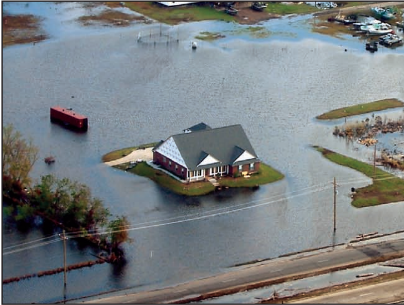
Figure 6-4. PLAQUEMINES PARISH, LOUISIANA: Home that had been elevated on fill, during the aftermath of Hurricane Katrina. (Source: FEMA 549)
