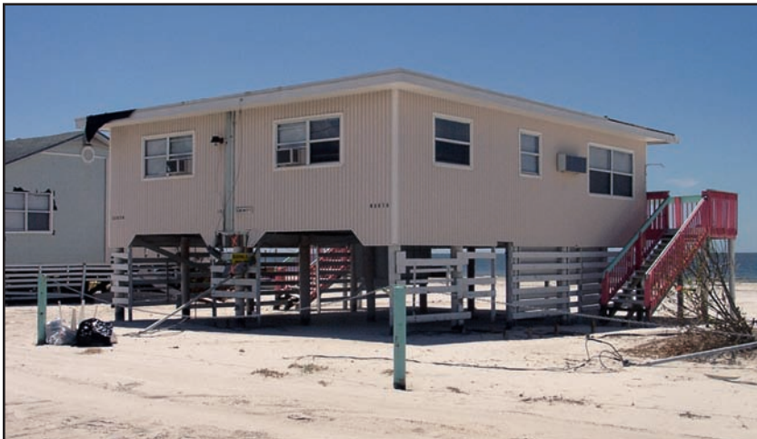
Figure 6-8. FORT MYERS BEACH, FLORIDA: Oceanfront house constructed on an open foundation sustained only minor damage after being exposed to high winds and storm surge. (Source: FEMA 488)
