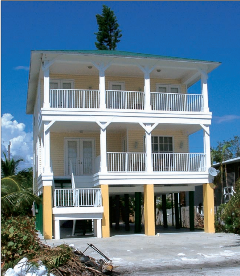
Figure 6-9. FORT MYERS BEACH, FLORIDA: Newly constructed house elevated on an open foundation sustained no storm surge damage when surges several feet deep impacted this site in 2004. (Source: FEMA 488)
