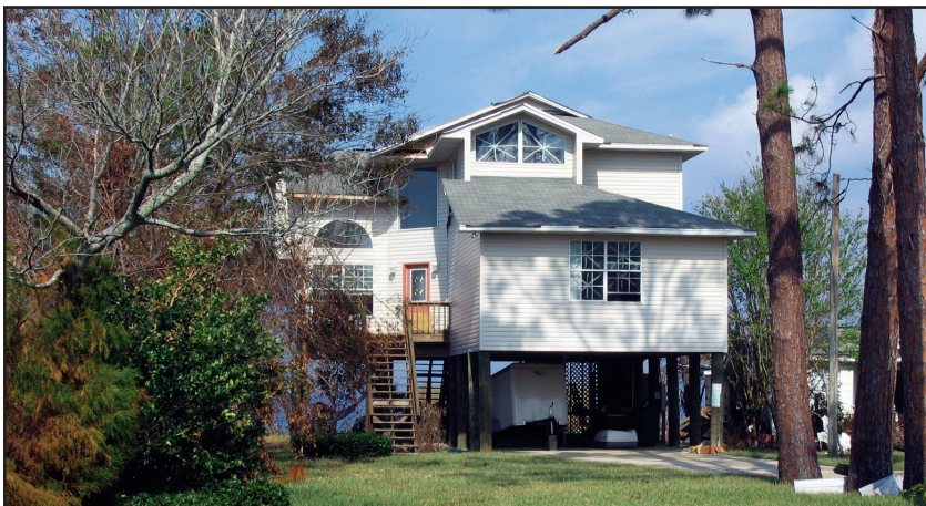
Figure 5-10. BIG LAGOON, FLORIDA: This house was elevated on piles, preventing severe damage from coastal flooding. (Source: FEMA 489)
