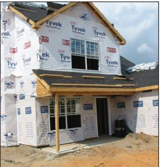
Figure 9-1 and 9-2. Examples of moisture barrier systems. (Source: FEMA 549)
