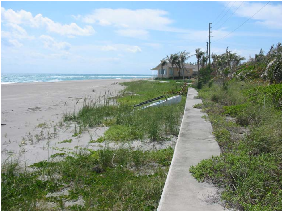
Figure D.2.10-4. Examples of a Buried Coastal Structure that Could Affect Flood insurance risk zones and BFEs
