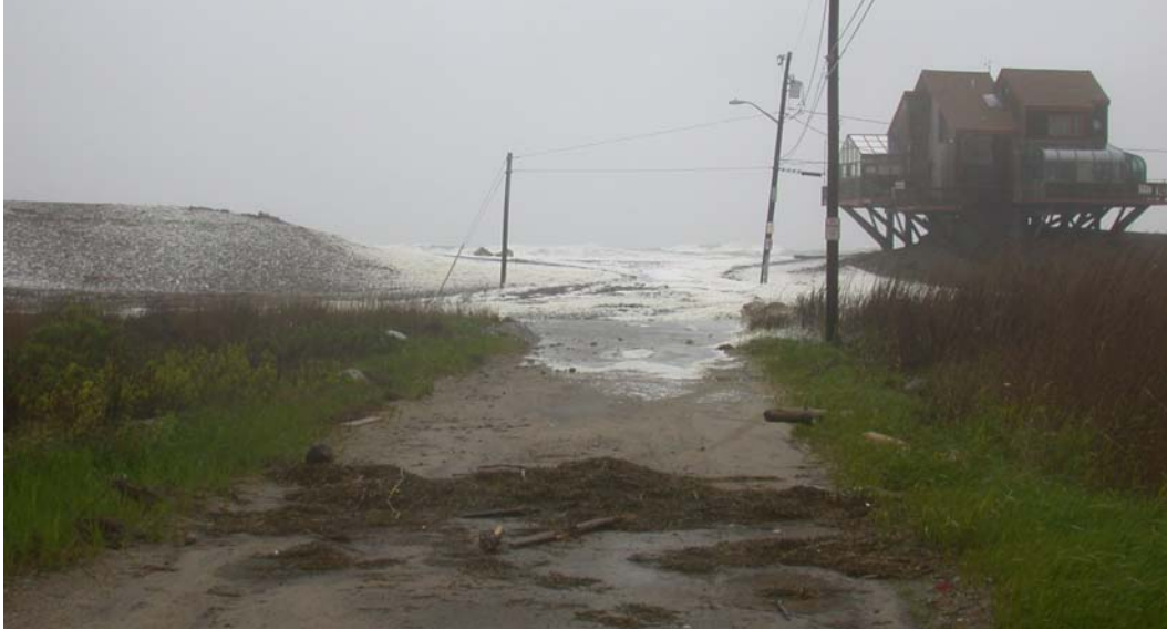
Figure D.2.9-17. Breach of mixed-sediment beach following a May 2005 northeaster, Mann Hill Beach, Massachusetts (Photo courtesy of R. Haney, Massachusetts Coastal Zone Management)
