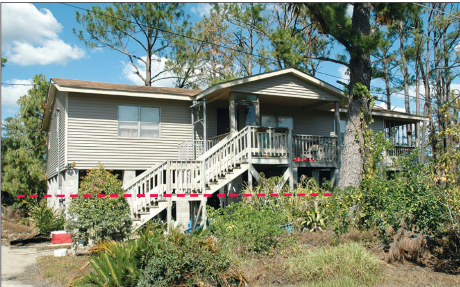
Figure 9-6. Another post-Katrina photo of an HMGP-elevated house. Note the estimated water line associated with Hurricane Katrina (red line) (Lacombe, Louisiana).
