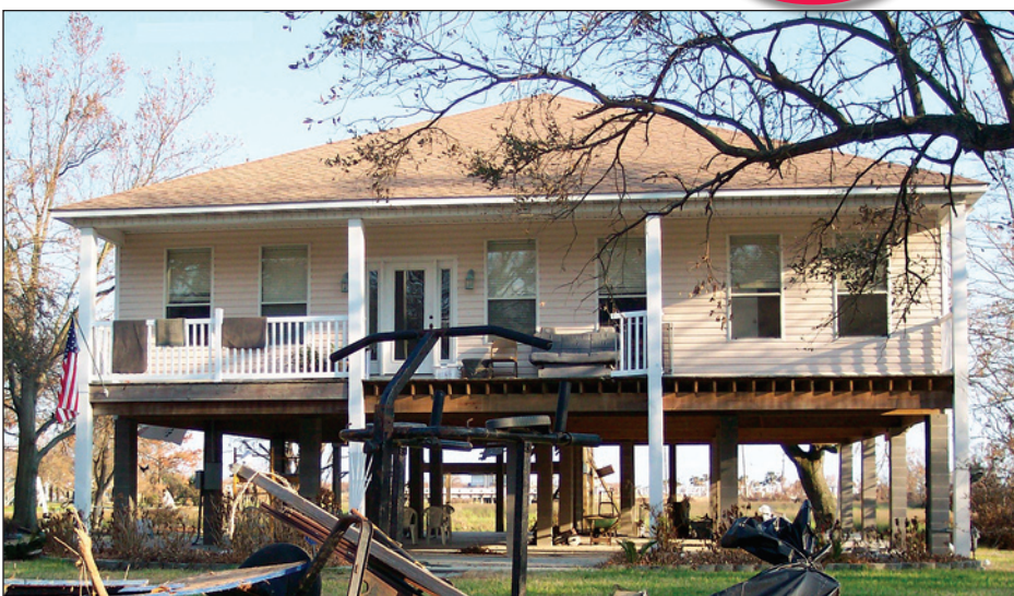
Figure 9-17. This photo was taken post-Katrina, illustrating the successful survival of this elevated building. The house was elevated to the citywide standard of 13.1’ msl using Increased Cost of Compliance funding (Pascagoula, Mississippi).
