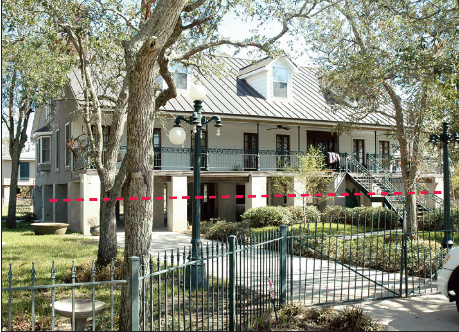
Figure 9-10. Another example of an elevated house that sustained only minor damage. Note the estimated flood depth in relation to the first floor (red line) (Mandeville, Louisiana).
