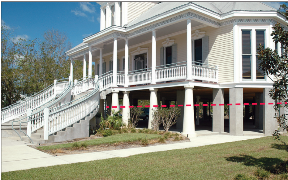
Figure 9-11. This building was relocated from New Orleans for use as a restaurant. The local building inspector recommended the elevation seen here, which protected this building from flood damage. Note the estimated flood depth in relation to the first floor (red line) (Mandeville, Louisiana).
