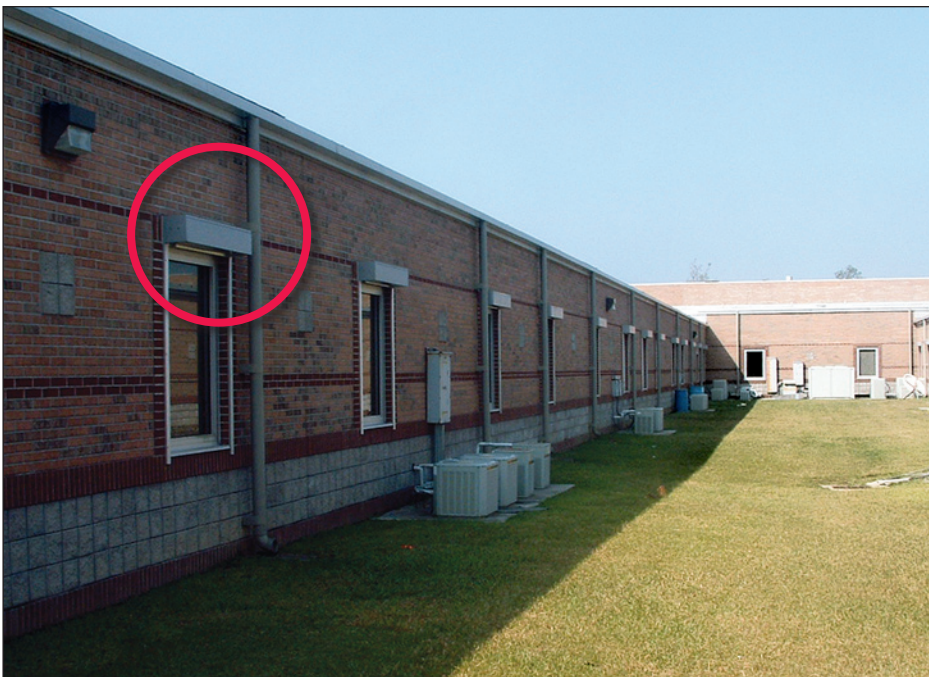
Figure 9-13. View of the Ocean Springs Middle School. Note the roll-down shutters over the windows (one example circled) (estimated wind speed: 120 mph. Ocean Springs, Mississippi).
