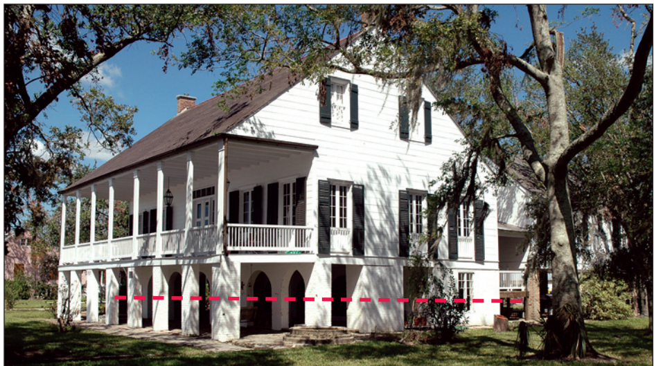
Figure 9-9. In contrast to the preceding examples, this 100-year-old building, also on the National Register of Historic Places and located next door to the house in Figure 9-7, received minimal damage. Note the estimated flood depth in relation to the first floor (red line) (Mandeville, Louisiana).
