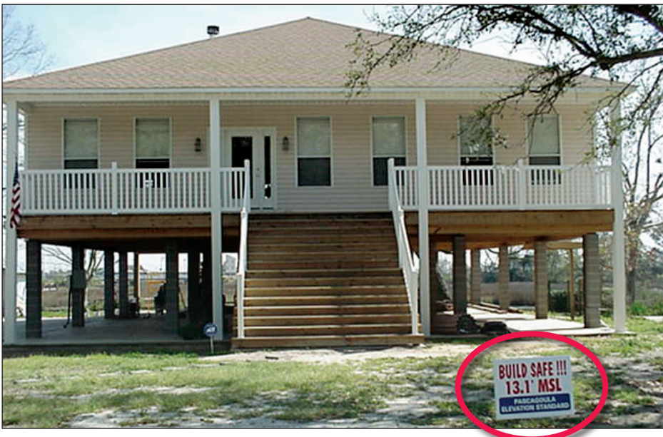
Figure 9-16. This photo was taken pre-Katrina ca. 1999/2000. Note the “Build Safe! 13.1’ MSL Pascagoula Elevation Standard” sign in front yard (circle) (Pascagoula, Mississippi).
