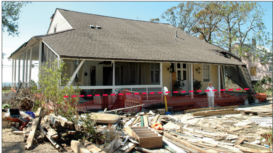
Figure 9-8. This building is the oldest house in Mandeville (built in 1836) and is on the National Register of Historic Places. The house is elevated 3 feet on piers and suffered wave damage to 18 inches above the floor. Note the estimated flood depth in relation to the first floor (red line) (Mandeville, Louisiana).
