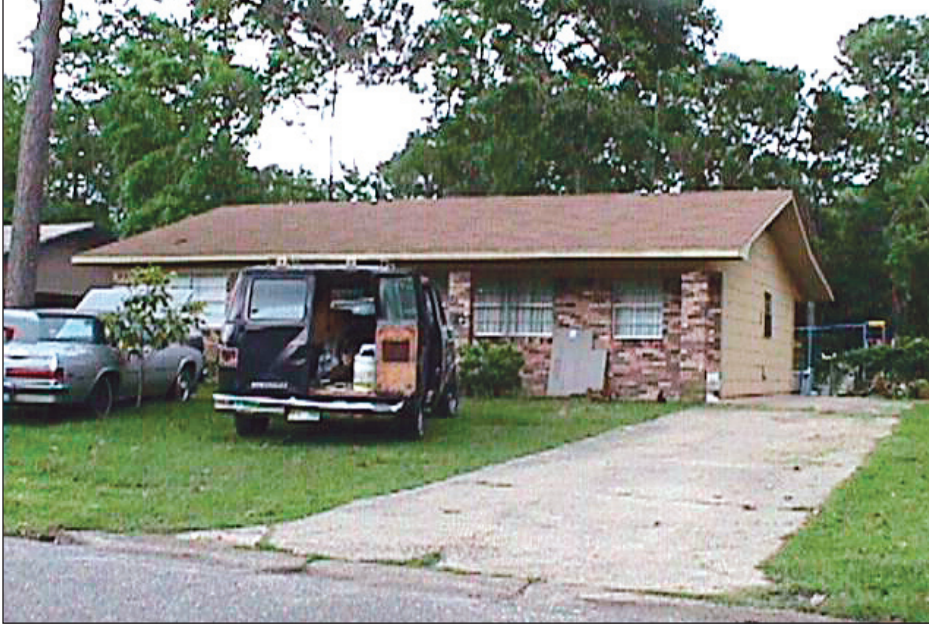
Figure 9-2. Pre-acquisition/pre-demolition photo of representative building included in project (photo ca. 1999/2000) (Gulfport, Mississippi)
