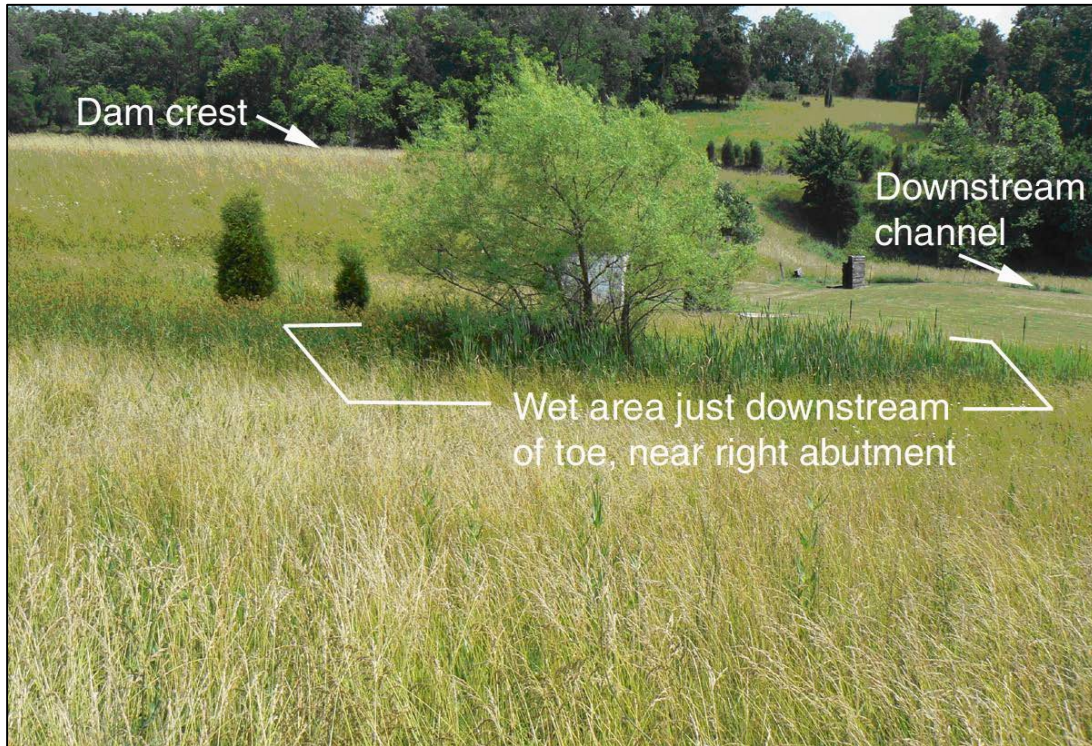
Figure 6-3.—Presence of phreatophytic vegetation (willow trees and cattails) in an established seepage discharge location approximately 200 feet below the downstream toe.
