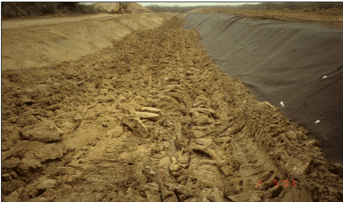
Figure 5.—Backfilling foundation trench, Olmitos-Garcias No. 2 Dam.
