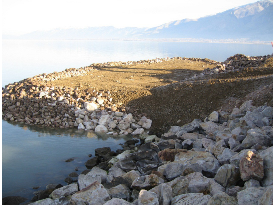
Figure 5.—Erosion into the South Drain did not stop until an upstream berm of gravel and pit-run material was pushed into reservoir.
