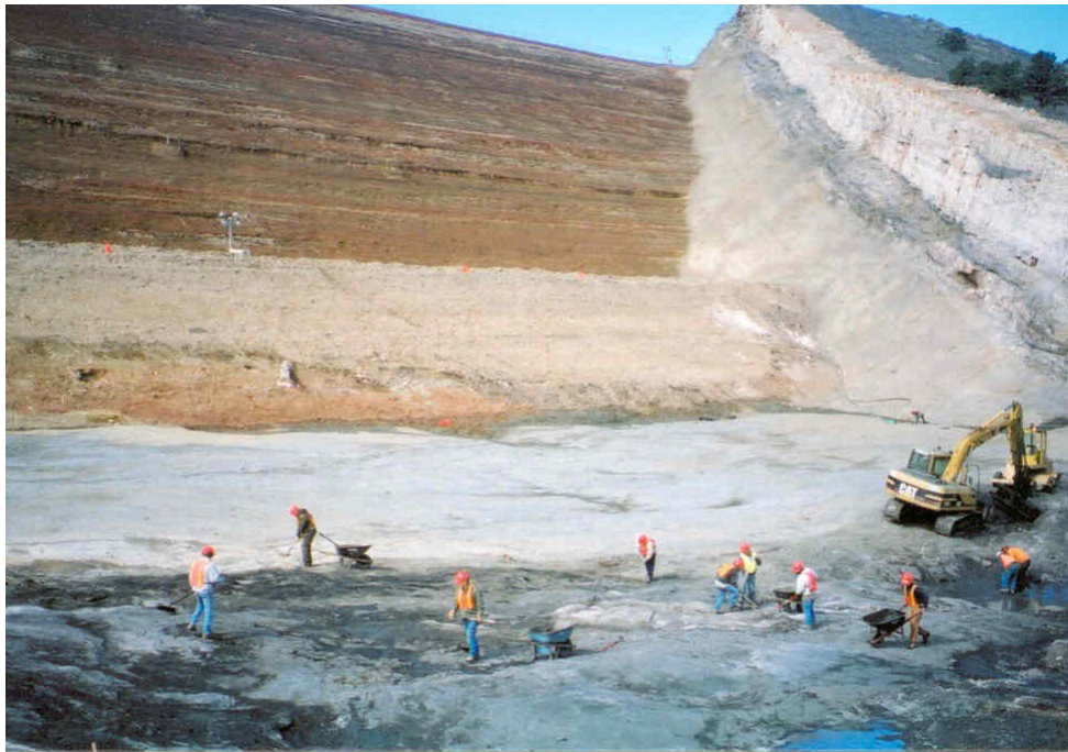
Figure 9.—Excavated downstream embankment and foundation at Soldier Canyon Dam.
