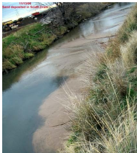
Figure 6-1.—Visual observation of failure mode in progress.
