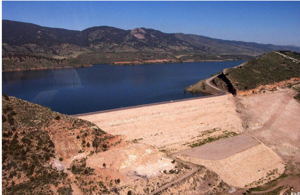
Figure 10.—Completed downstream modification at Dixon Canyon Dam.
