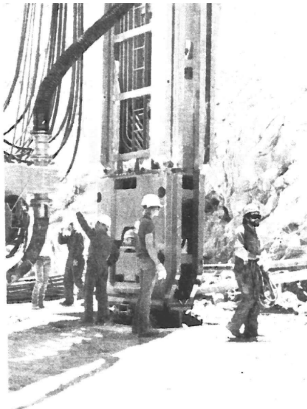
Figure 4.—View of Hydrofraise being maneuvered and lowered for panel excavation.
