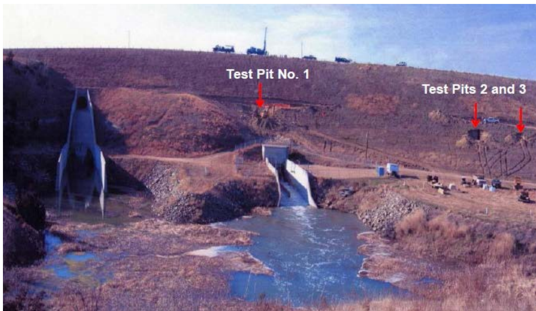
Figure 4.—Photo showing locations of observed cracking in the embankment.
