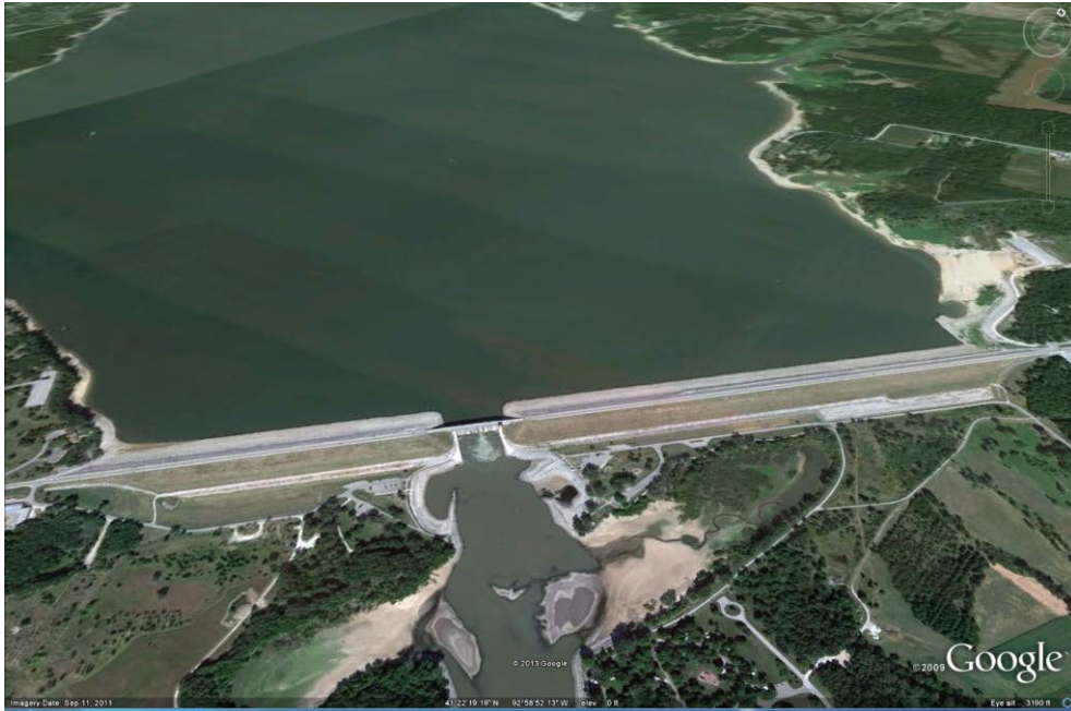
Figure 1.—Oblique view of Red Rock Dam (Google Earth, September 11, 2011).
