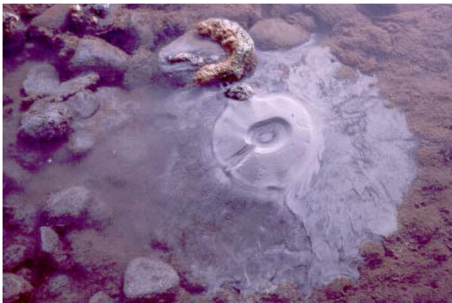
Figure 2.—Boils in outlet channel at Canby Creek, R-1 Dam, Minnesota.
