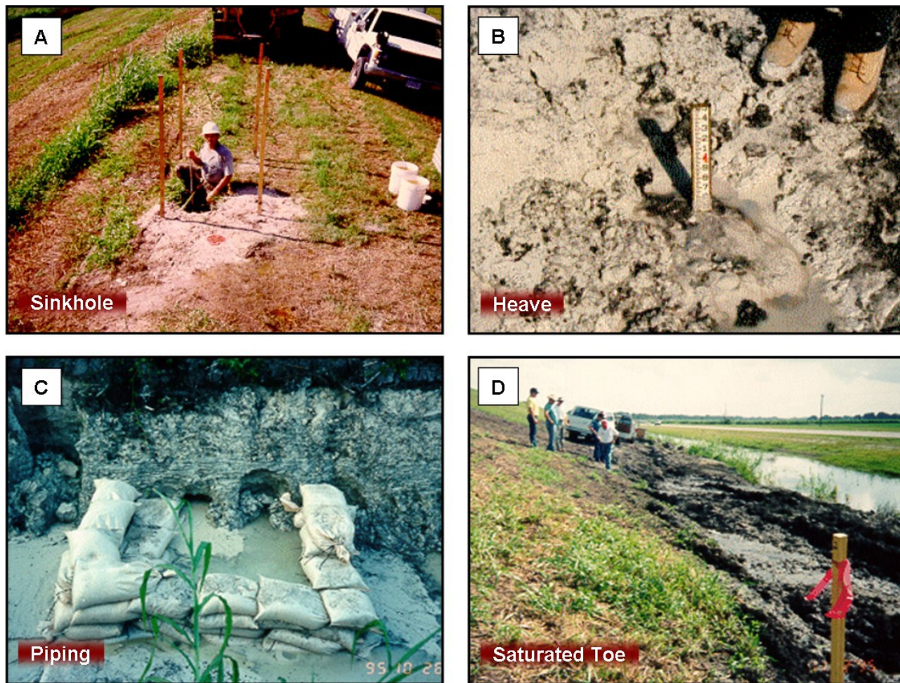
Figure 3.—Representative photographs of prior seepage erosion conditions at HHD near Lake Harbor. Downstream area seepage distresses were observed during events having a ~30-yr return period: (A) sinkhole formation in crest, (B) heave of downstream toe caused by upward seepage flow - surveyrod was easily embedded 4 ft deep, (C) piping at downstream toe of dike, and (D) saturation of landward toe and embankment slope.
