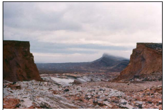
Figure 1b.—Breach through Quail Creek Dike.
