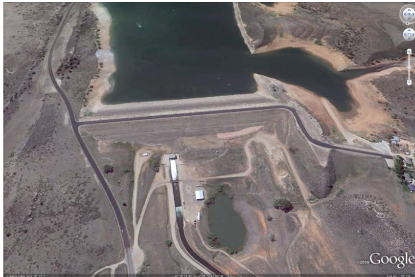
Figure 2.—Oblique view of Horsetooth Dam and Satanka Dike (looking south).
