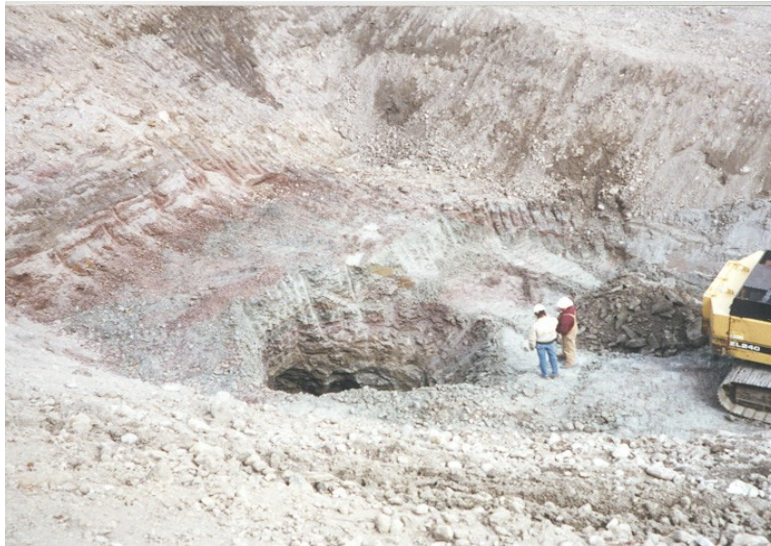
Figure 3.—View from top of dam after excavation was complete.
