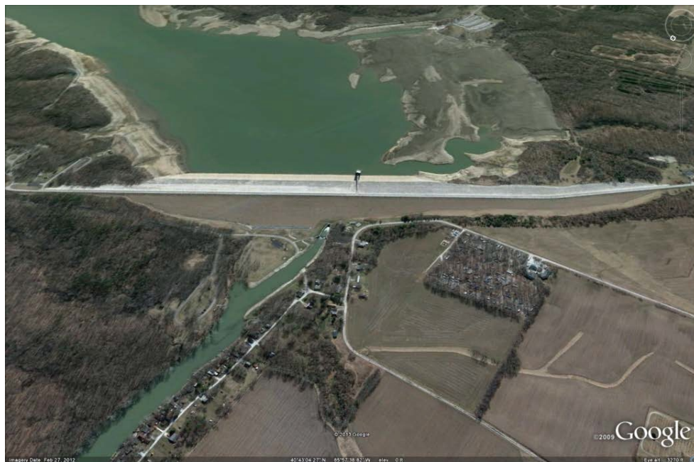
Figure 2.—Oblique view of dam (Google Earth, February 27, 2012).
