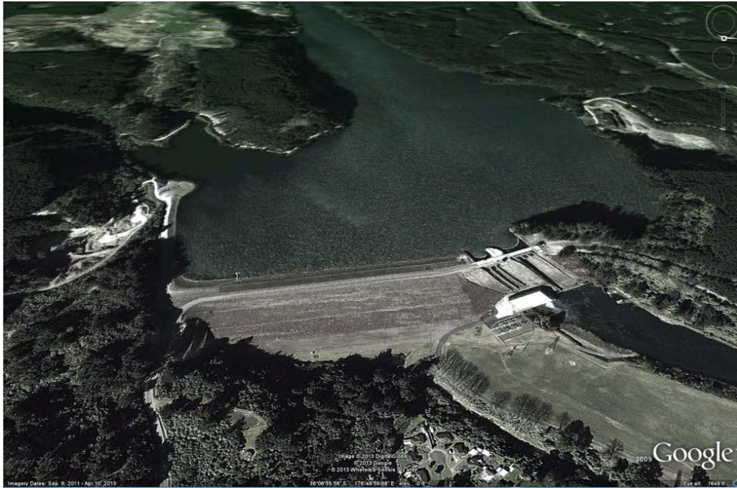
Figure 1.—Oblique view of Matahina Dam (Google Earth, September 9, 2011).
