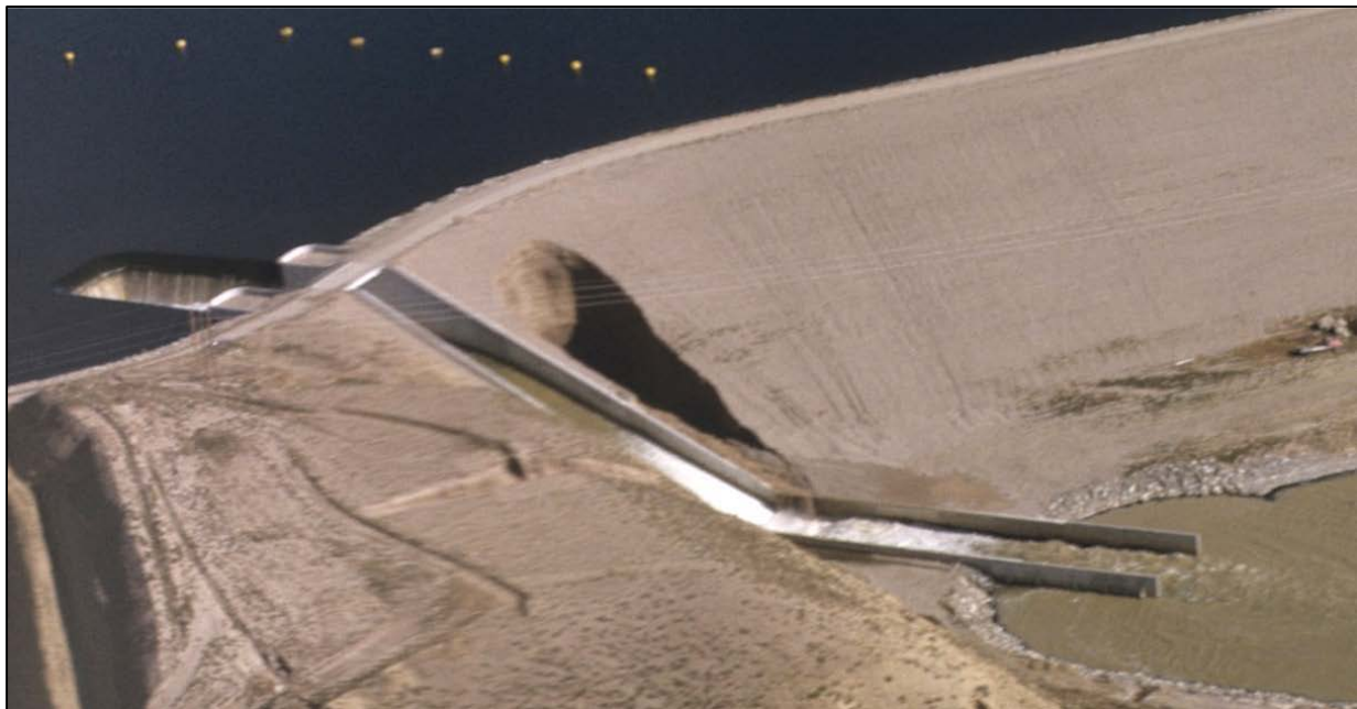
Figure 4-7.—Fontenelle Dam, which nearly breached by sloughing.
