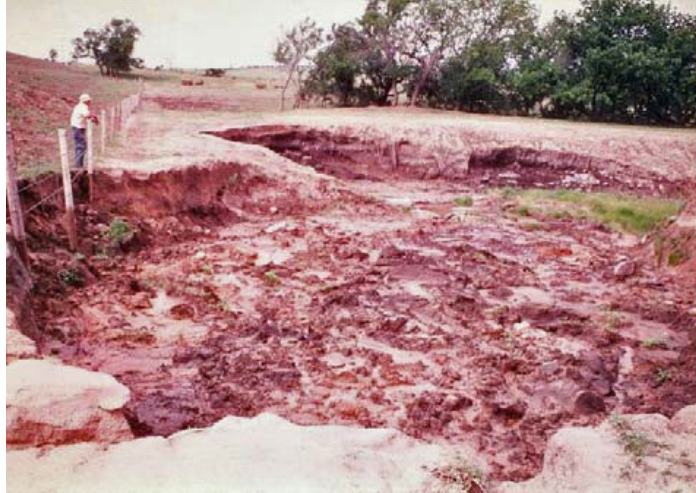
Figure 4.—Sloughing of downstream area observed in May 1979.
