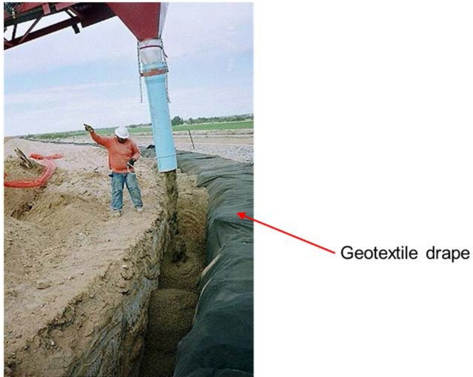
Figure 5.—Placing filter material with tremie, Florence Dam.
