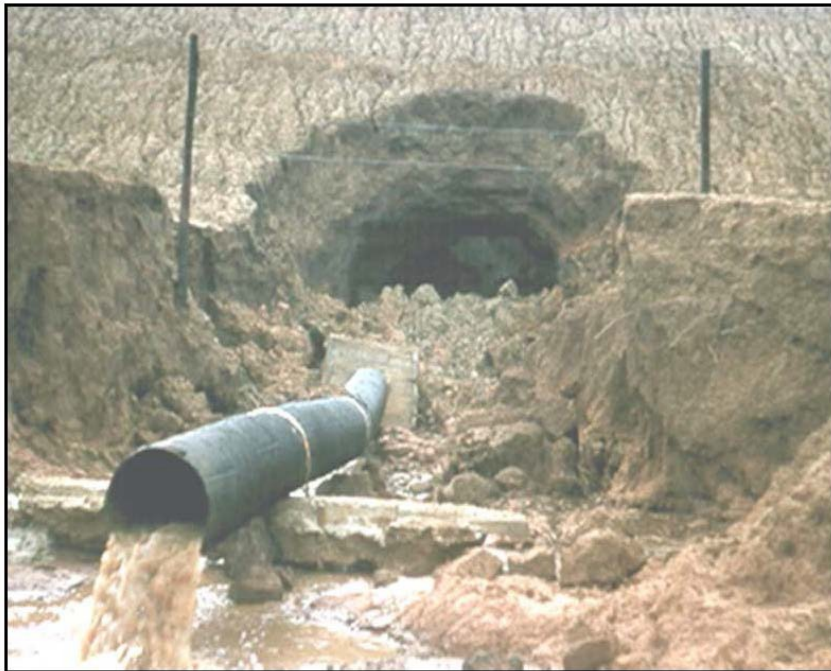
Figure 4-6.—Example of a dam that experienced gross enlargement, but the reservoir drained before erosion progressed to the point of crest collapse.
