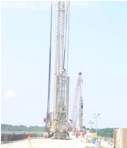
Figure 9.—Typical hydromill configuration.
