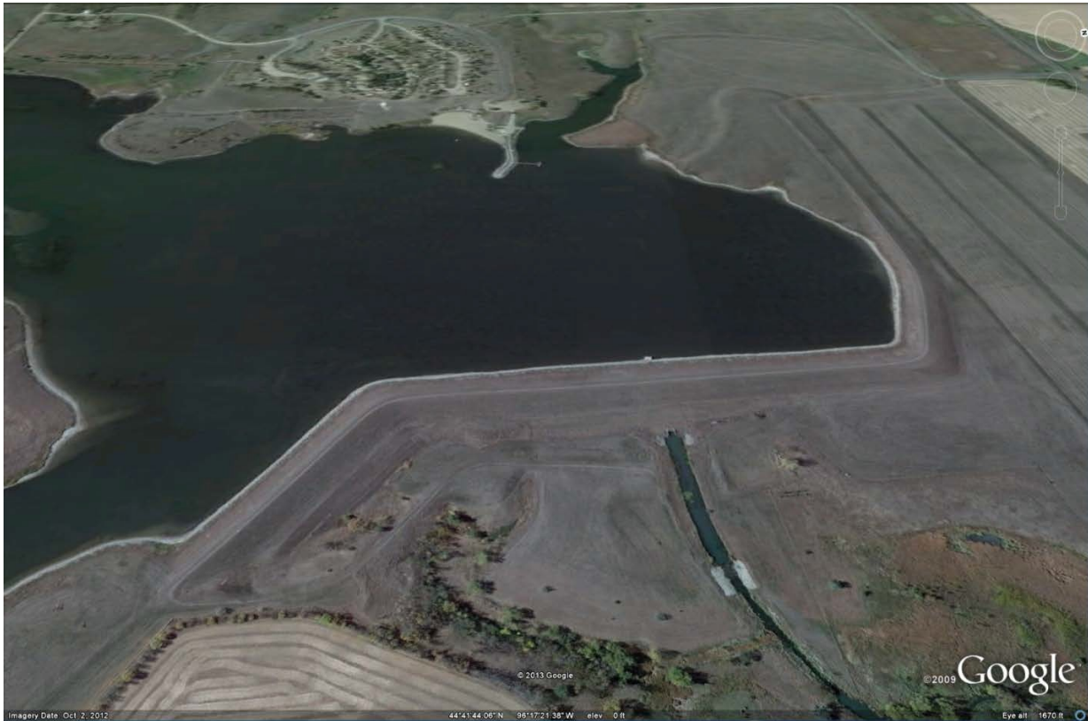
Figure 1.—Oblique view of Canby Creek, R-1 Dam (Google Earth, October 2, 2012).
