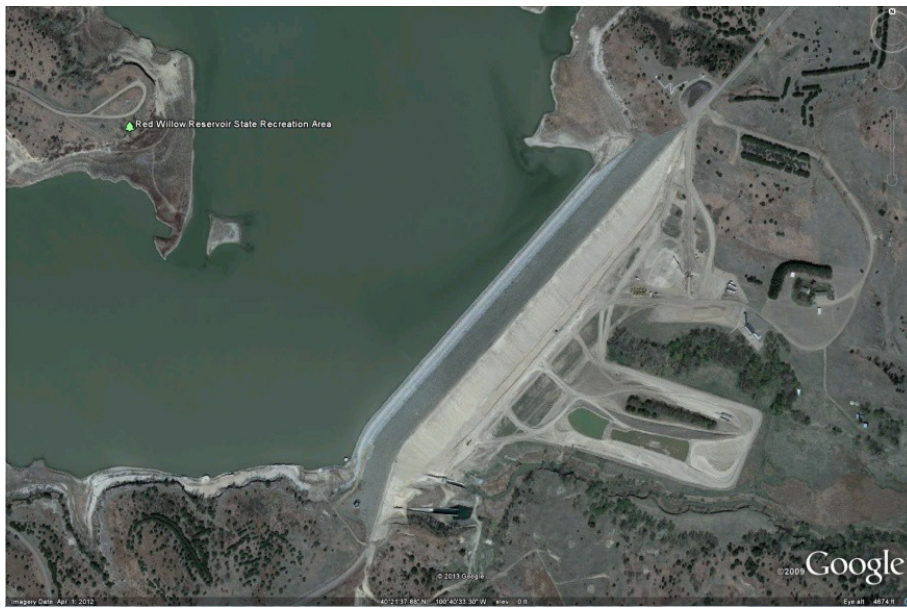
Figure 1.—Red Willow Dam.
