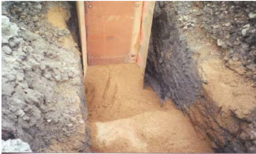
Figure 3.—Trench drain installation at Canby Creek, R-1 Dam.
