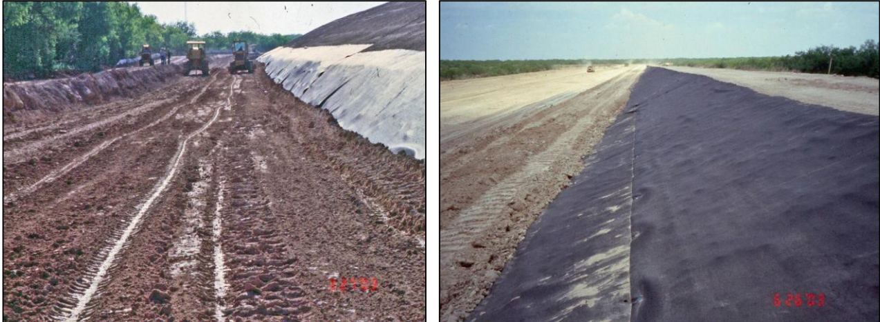
Figure 10-18.—Construction of geotextile barrier in Olmitos-Garcias No. 2 Dam in south Texas. The downstream side of the embankment is shown. Left – geotextile being backfilled in foundation trench. Right – geotextile on back slope of dam prior to backfilling. (Photos courtesy of NRCS, Texas)
