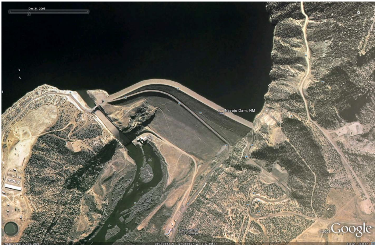
Figure 1.—Navajo Dam and spillway (Google Earth, June 30, 2005).
