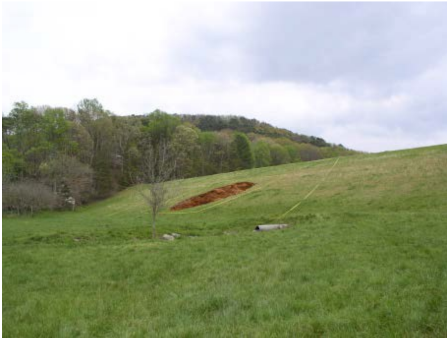
Figure 4-9.—Sallacoa Dam experienced a large sinkhole from internal erosion into a karst foundation.
