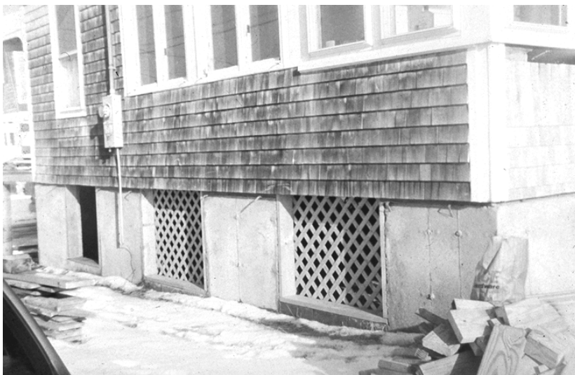
Figure 5-10: Building elevated on crawlspace with openings.
