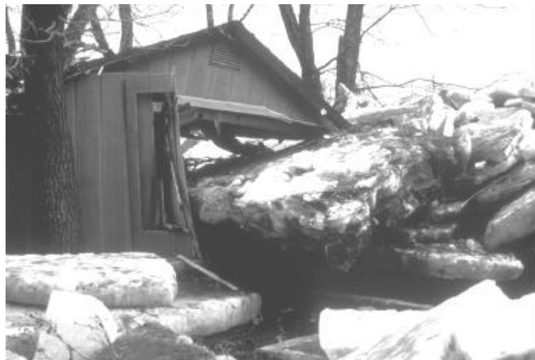
Figure 1-18. Ice floes and other large items of debris can crush a house
