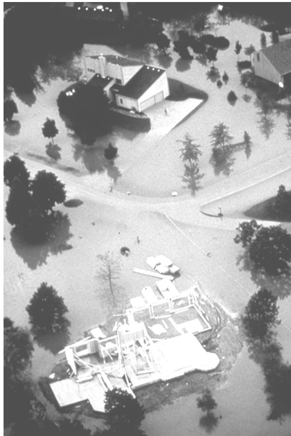
Figure 5-7. These two new buildings elevated on fill were not damaged by this 100-year flood.
