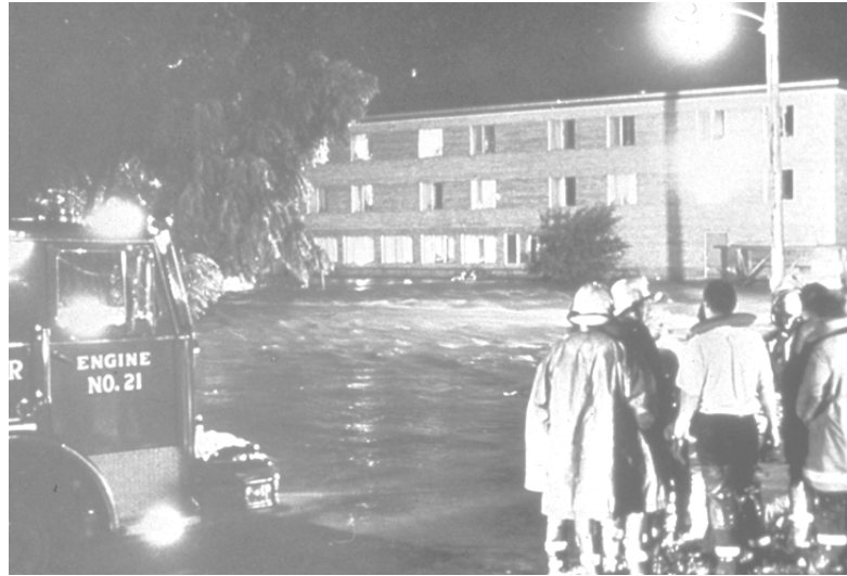
Figure 6-4: Four people died in a 1978 flood in this critical facility. This nursing home in Rochester, Minnesota, was isolated by high velocity floodwaters. Because there was no dry land access, firefighters could not rescue the occupants.
