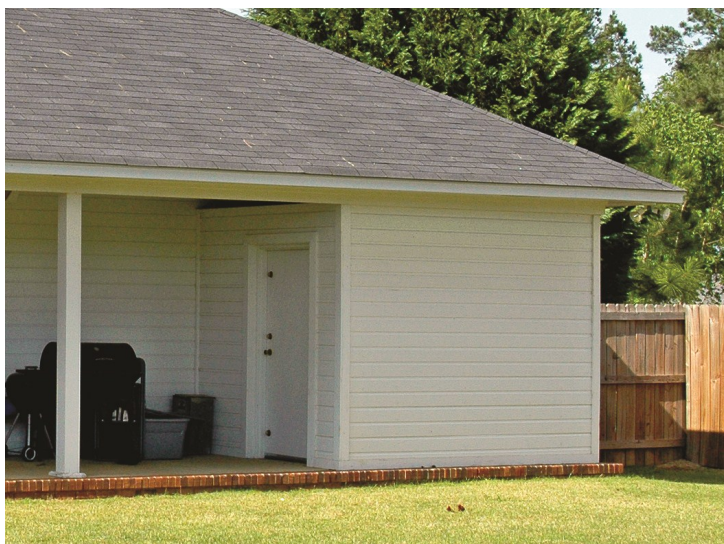
An above-ground safe room constructed as an addition to a slab-on-grade home in a way that matches the aesthetics of the home (Tuscaloosa, AL).
