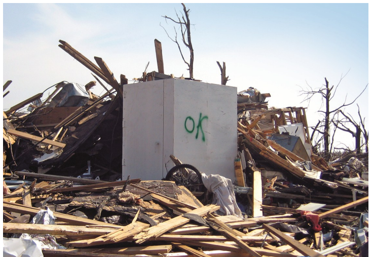
Above-ground residential safe room that was in the garage of a home hit by an EF5 tornado (Joplin, MO).
