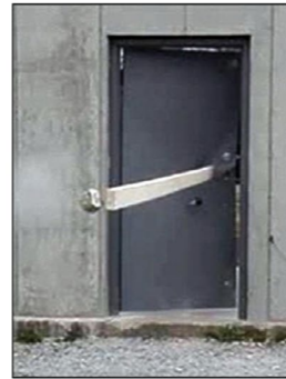
Tornado safe room impact test results: Door assembly failed at latch/lock
