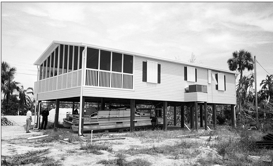
Figure 8-4. Manufactured home on a pile foundation.
