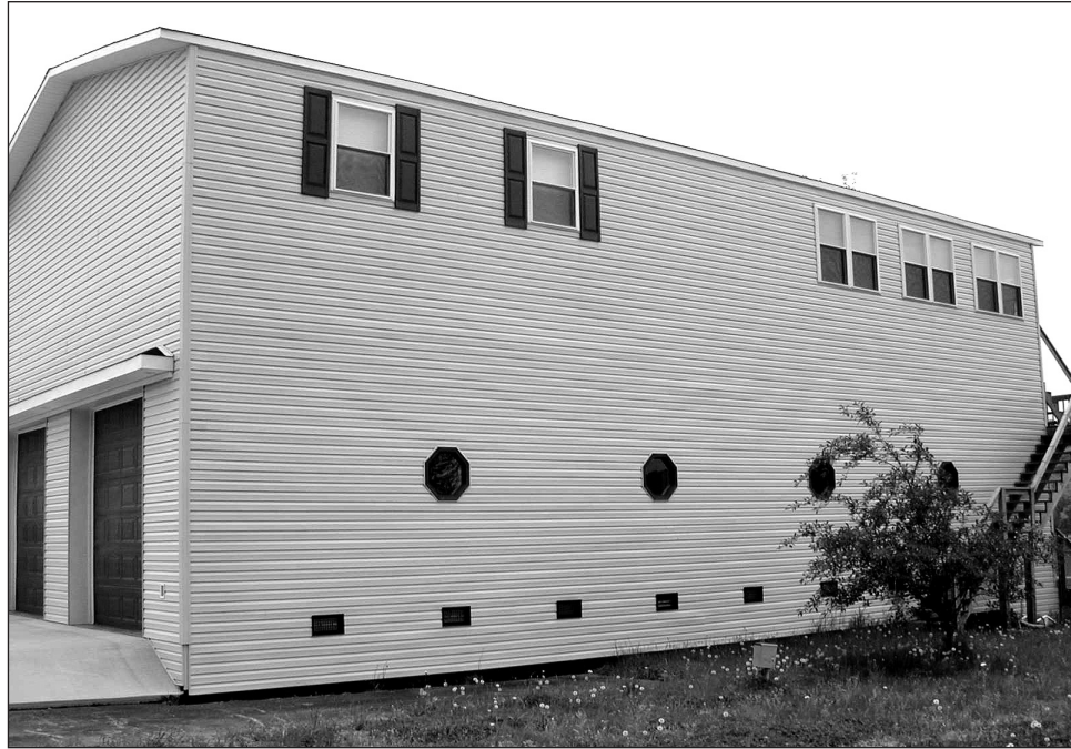
Figure 8-1. A manufactured home elevated on a perimeter foundation wall. Although it appears the openings are too high, the bottoms of the openings are less than 1 foot above the top of the interior slab.
