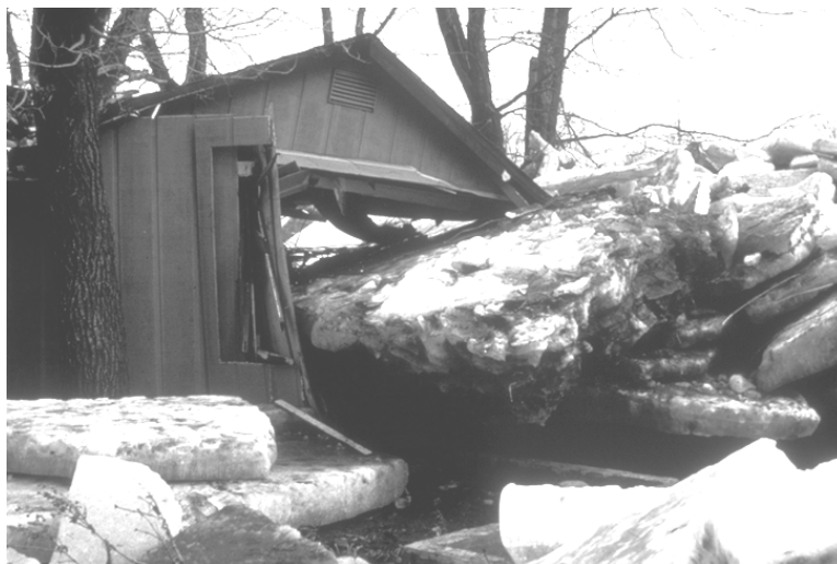
Figure 1-18. Ice floes and other large items of debris can crush a house
