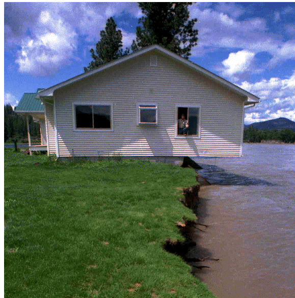
Figure 1-5. Riverine erosion can undercut structures
