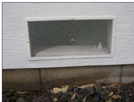
Figure 1. A closed foundation with a cripple wall (FEMA field team).
