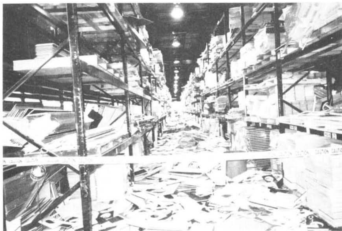
Damage to inventory on industrial storage racks Earthquake Damage: 1994, Northridge, California Photo Credit: Wiss, Janney, Elstner Associates, Inc.
