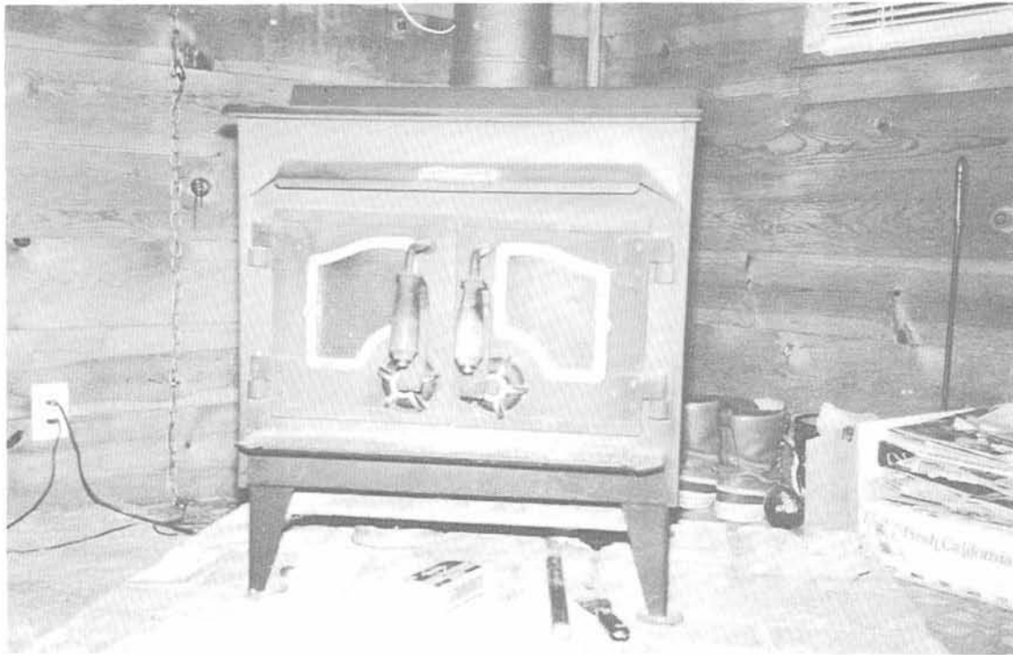
Unrestrained wood burning stove Photo Credit: Wiss, Janney, Elstner Associates, Inc.
