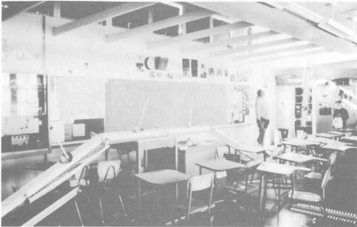
Failure of light fixtures at Northridge Junior High School Earthquake Damage: 1994, Northridge, California Photo Credit: Earthquake Engineering Research Institute, Gary L. McGavin
