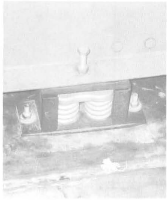
Chiller mount with no uplift resistance and insufficient or no shear resistance. Photo Credit: Wiss, Janney, Elstner Associates, Inc. Schematic Upgrade Detail: See Detail U32, Air Compressor
