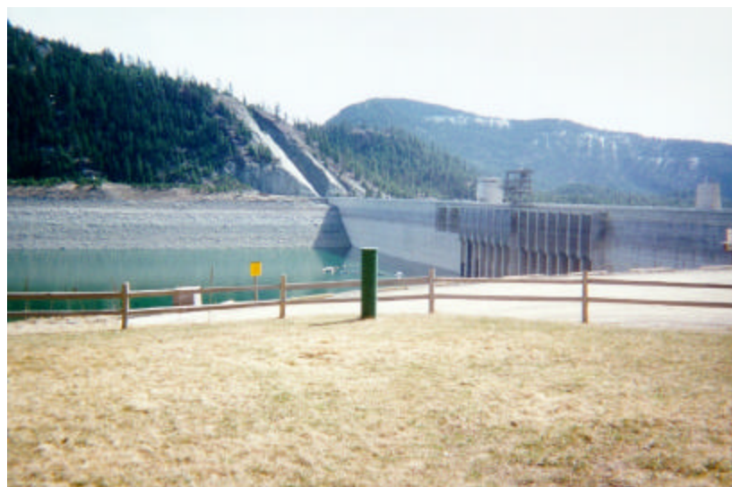
Figure C-4. Reference Station (R2), Libby Dam.
