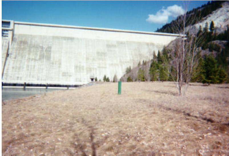
Figure C-5. Existing survey station, Libby Dam.
