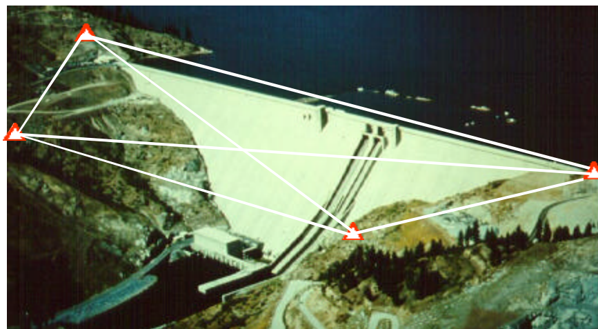
Figure 2-3. Reference network configuration for a concrete dam depicting reference points near abutments and at downstream locations
