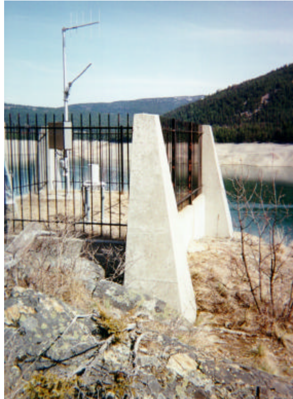
Figure C-3. Reference Station (R1), Libby Dam.
