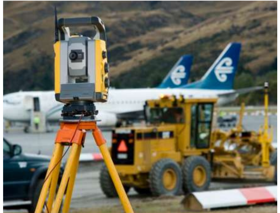
Pictures Provided by Jason Billerbeck of Peterson Contractors Inc.
