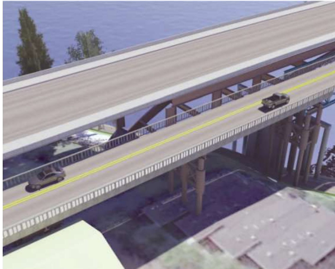
Traffic on detour bridge during construction of new bridge
