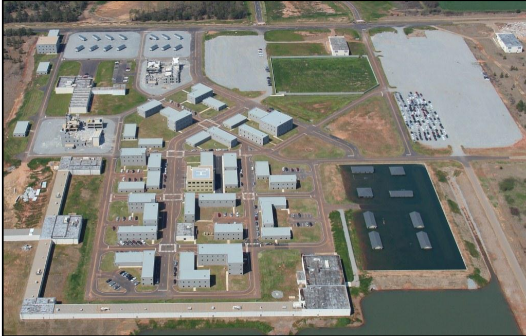
Figure 26. An Aerial Photograph of Guardian Centers Located in Perry, Georgia
