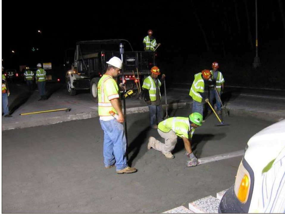
Figure 42. Base preparation and grading No. 10 aggregate for PPCP installation.
