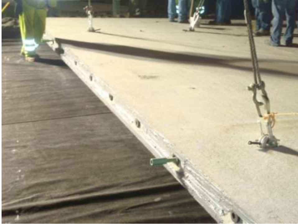
Figure 14. Ducts for post-tensioning strands.
