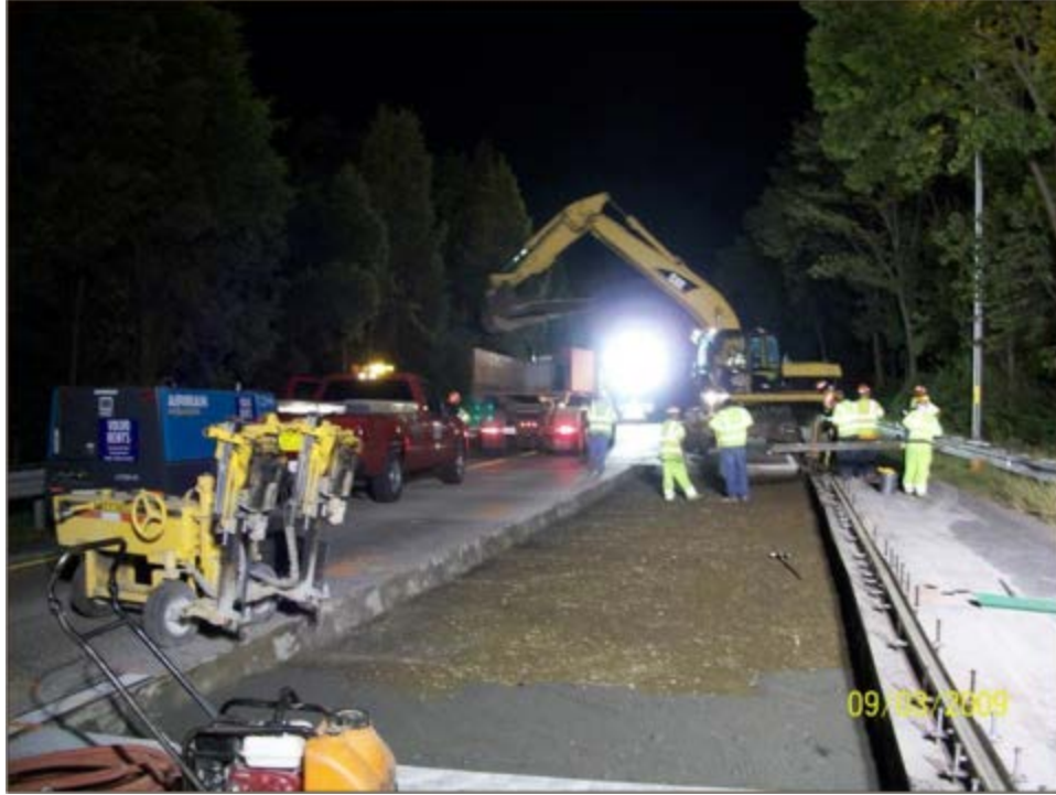
Figure 54. Removal of existing slab along ramp for Super-Slab ® installation.
