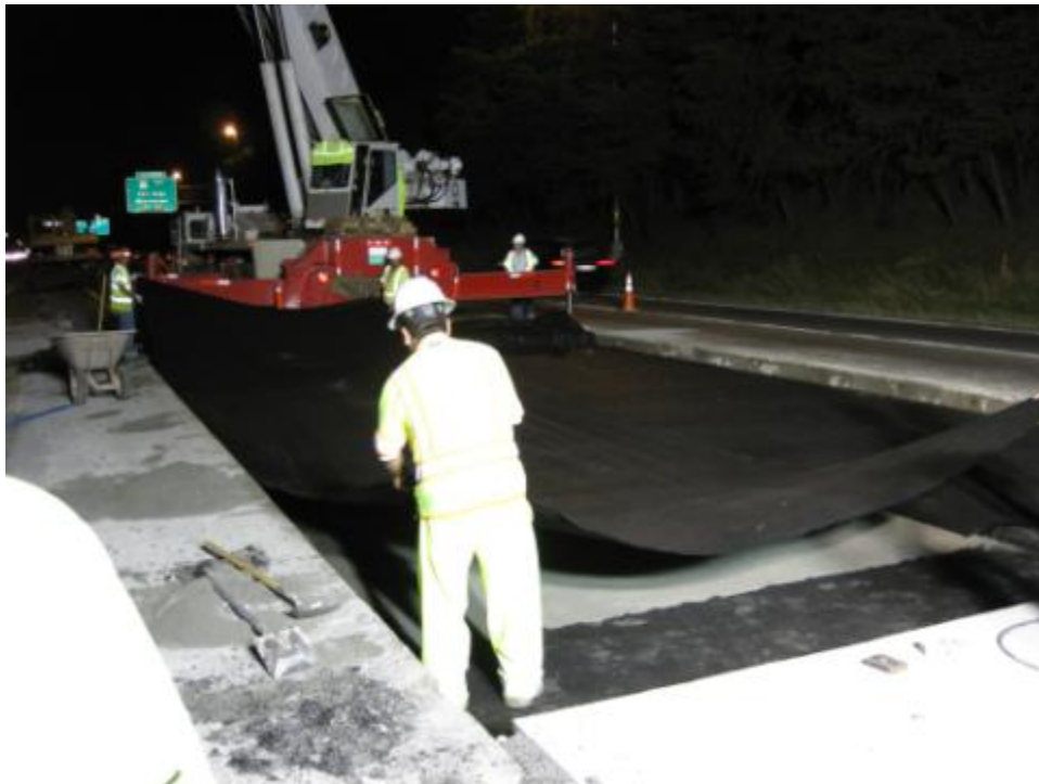
Figure 43. Geotextile fabric spread on graded base material to reduce slab-subbase friction.
