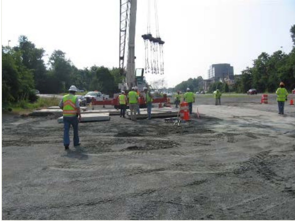
Figure 27. Trial installation for the PPCP system.
