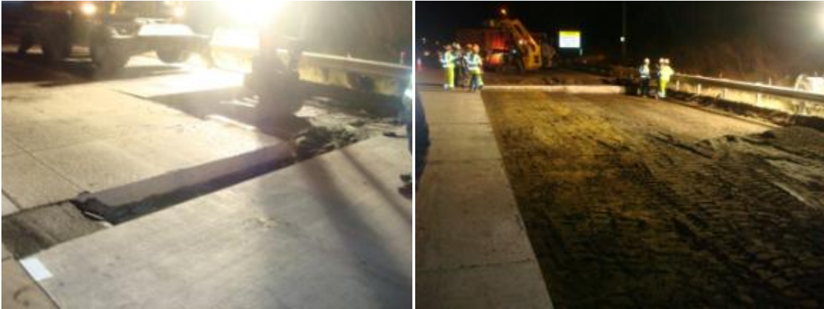
Figure 41. Removal of existing slabs.
