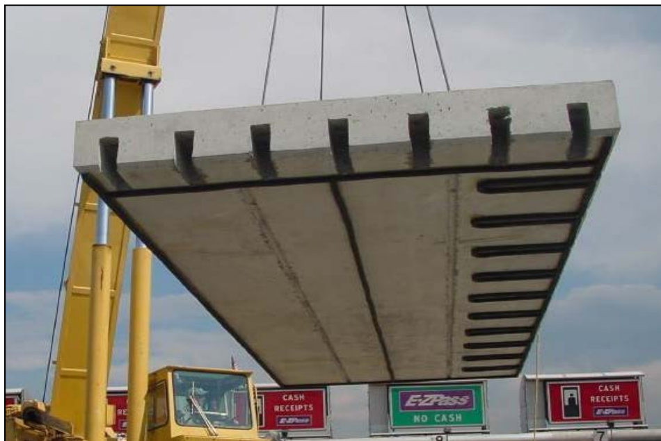
Figure 22. Grout distribution channel and foam gasket for bedding grout (image from project in New York State, 2002).
