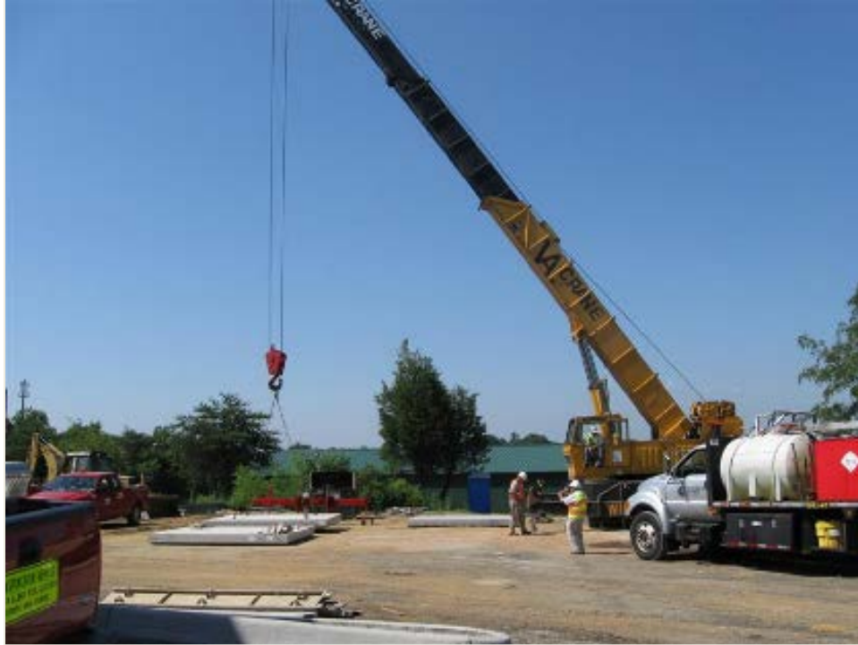
Figure 26. Trial installation for Super-Slab ® .
