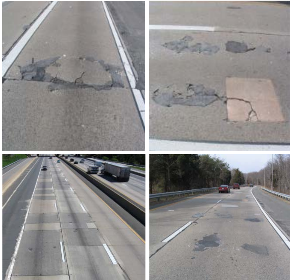
Figure 6. Surface condition of I-66 mainline and ramp leading to US 50 West in 2008.
