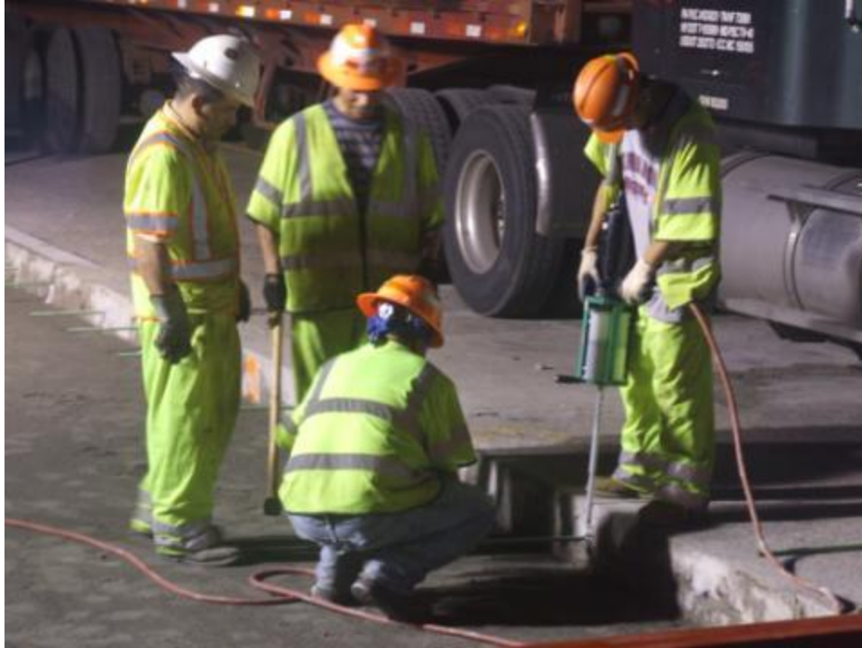
Figure 56. Anchoring tie bars in existing pavement in adjacent lane.
