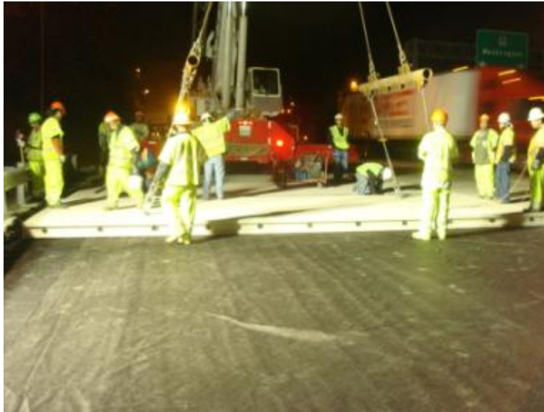
Figure 44. Slab placement and alignment (top and bottom).
