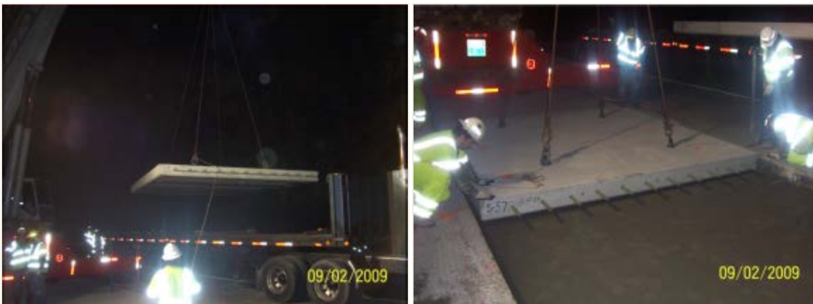
Figure 57. Slab installation.
