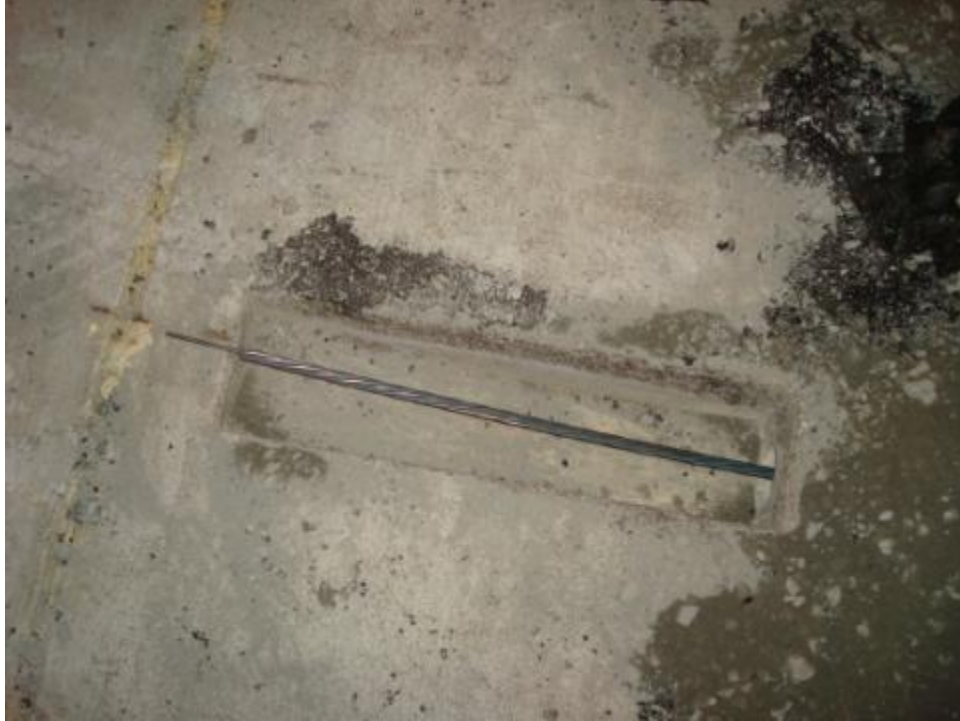
a) Tendon inserted in anchor panel blockouts
