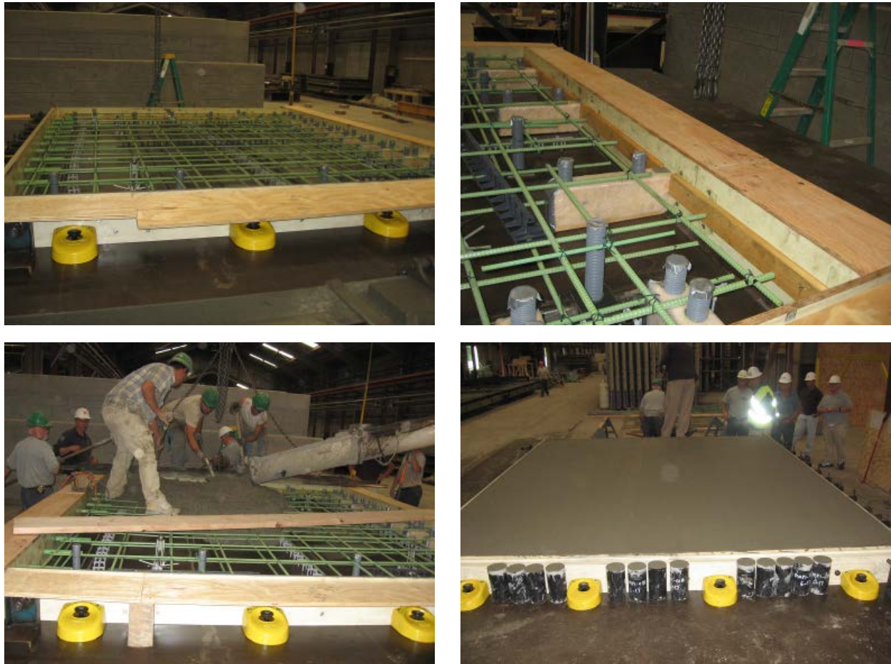
Figure 30. Precasting operations and form work details for the Super-Slab ® .
