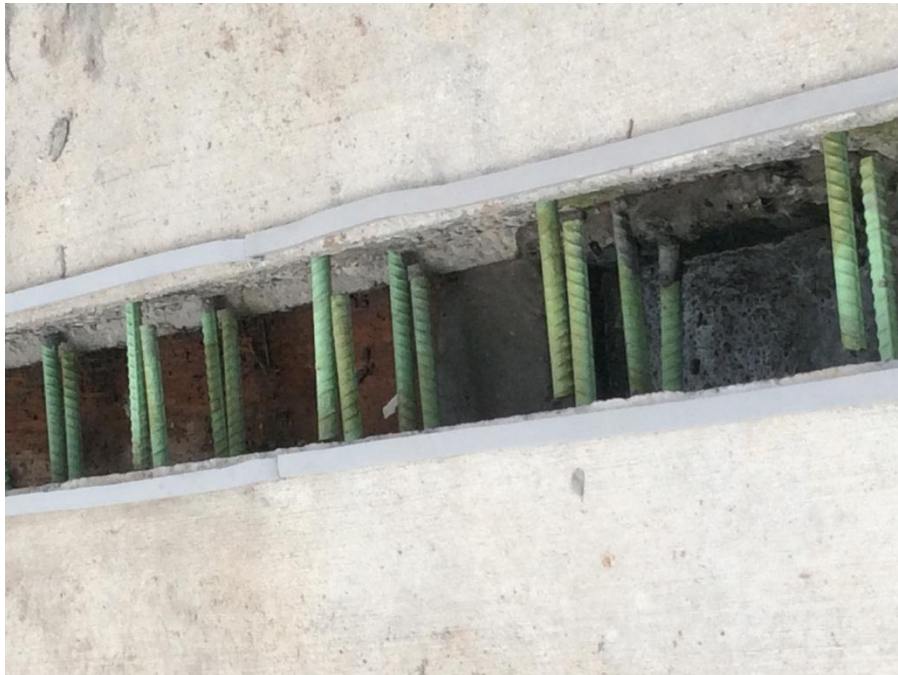
Figure 11. Photo. Transverse Deck Joint. (courtesy: UDOT)
