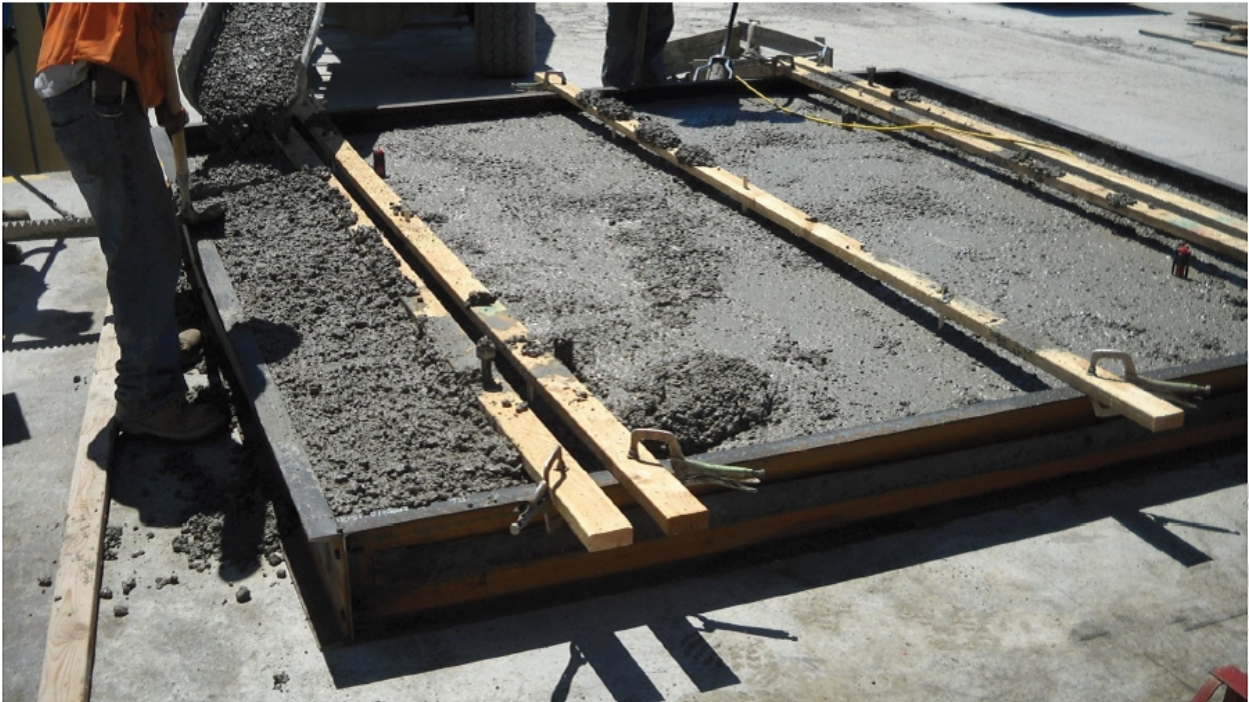
Figure 15. Pouring concrete in form to precast the panel.
