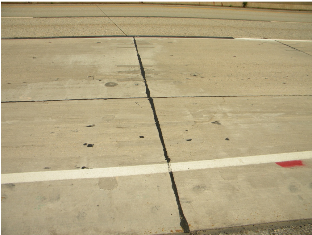
Figure 31. Transverse joint with grout-filled dowel bar slots.
