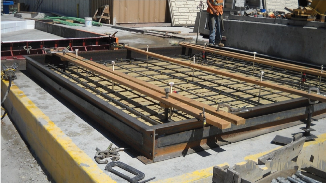
Figure 14. Completed form ready for concrete pour.
