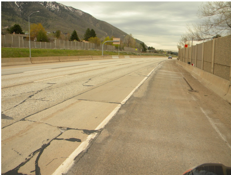
Figure 3. Southbound project view showing three lanes, merge area, and shoulder.
