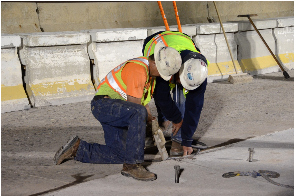
Figure 27. Placing preformed strip seal to contain grout.
