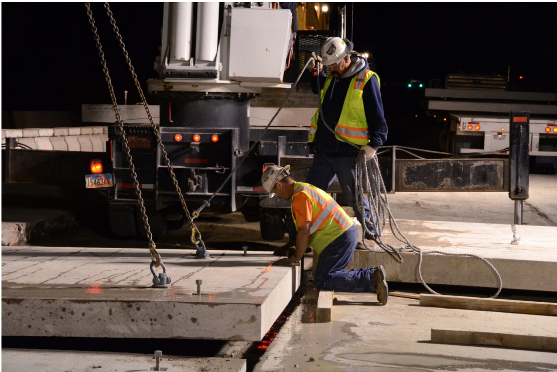
Figure 23. Steering precast panel into place onto the prepared base.
