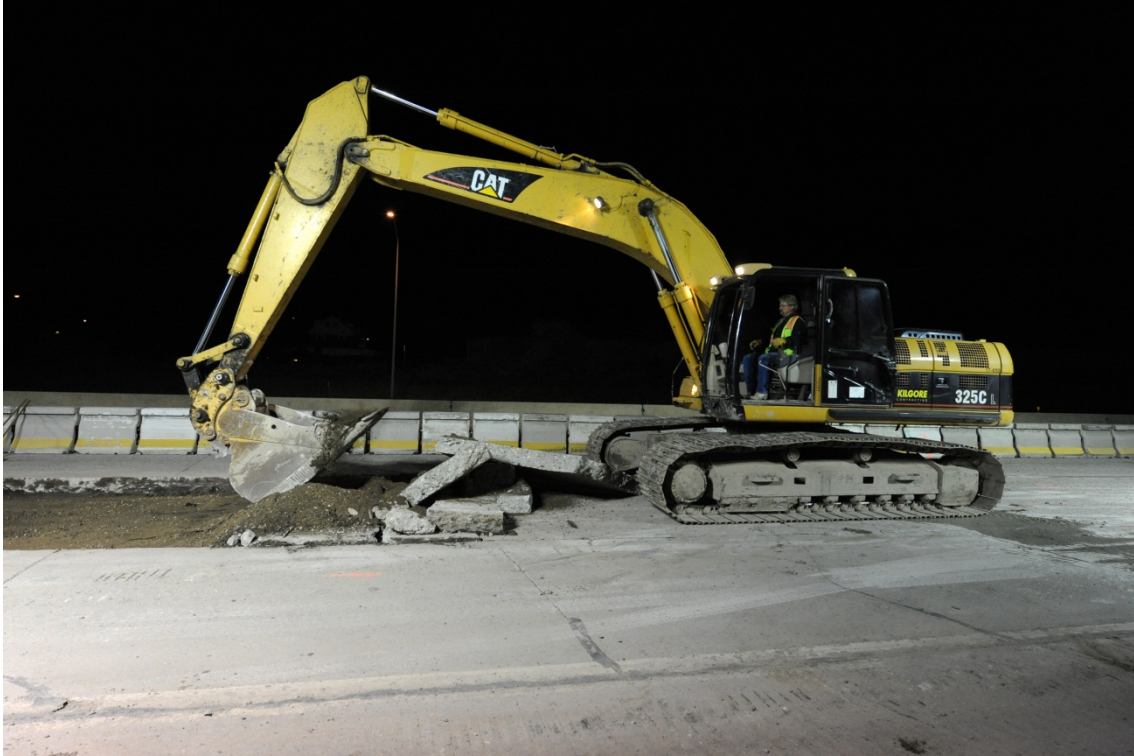
Figure 18. Removal of existing deteriorated pavement (lane 3).
