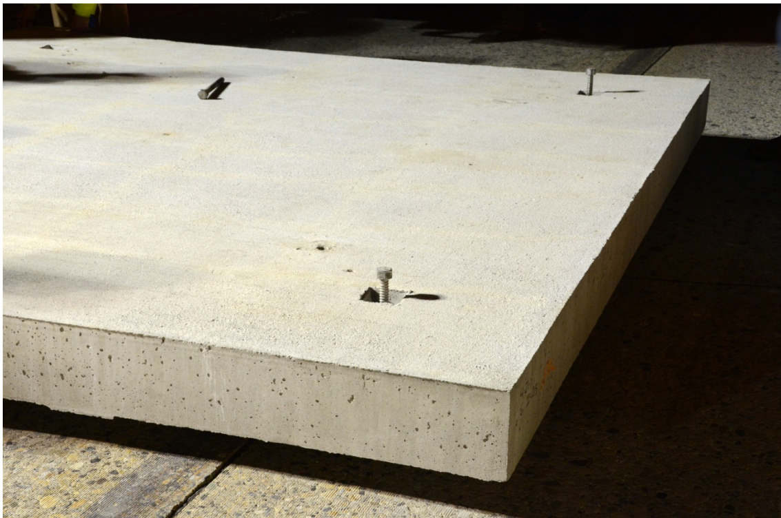
Figure 25. Leveling bolts used to level the panels on the leveling plates.
