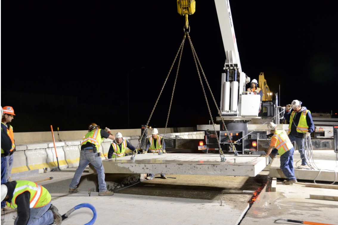
Figure 22. Placement of precast panel on the prepared base.
