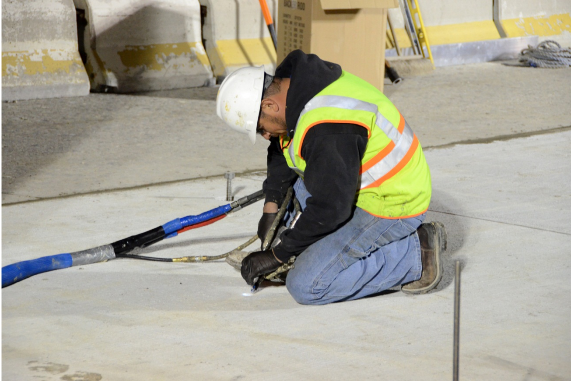
Figure 28. Urethane grout injected through the grout injection hole.
