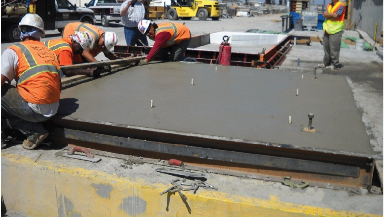
Figure 16. Removal of grout tube and bolt locator jigs.
