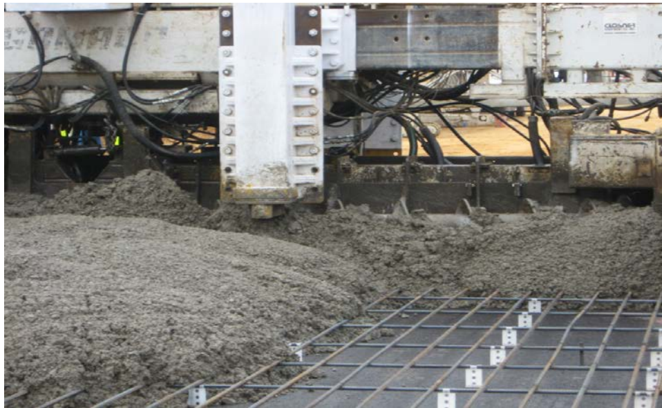
Figure 6. Optimized Aggregate Mix Placed in Front of Paver (Courtesy TxDOT)
