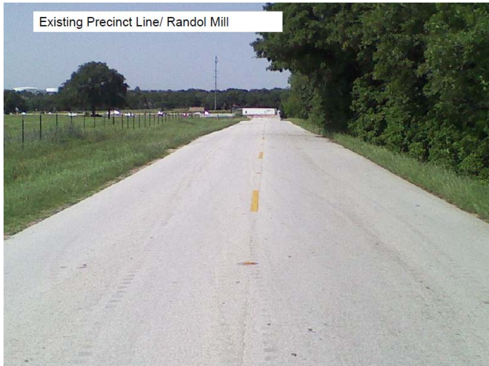
Figure 3. Existing Two-Lane Facility, Precinct Road (Courtesy TxDOT)
