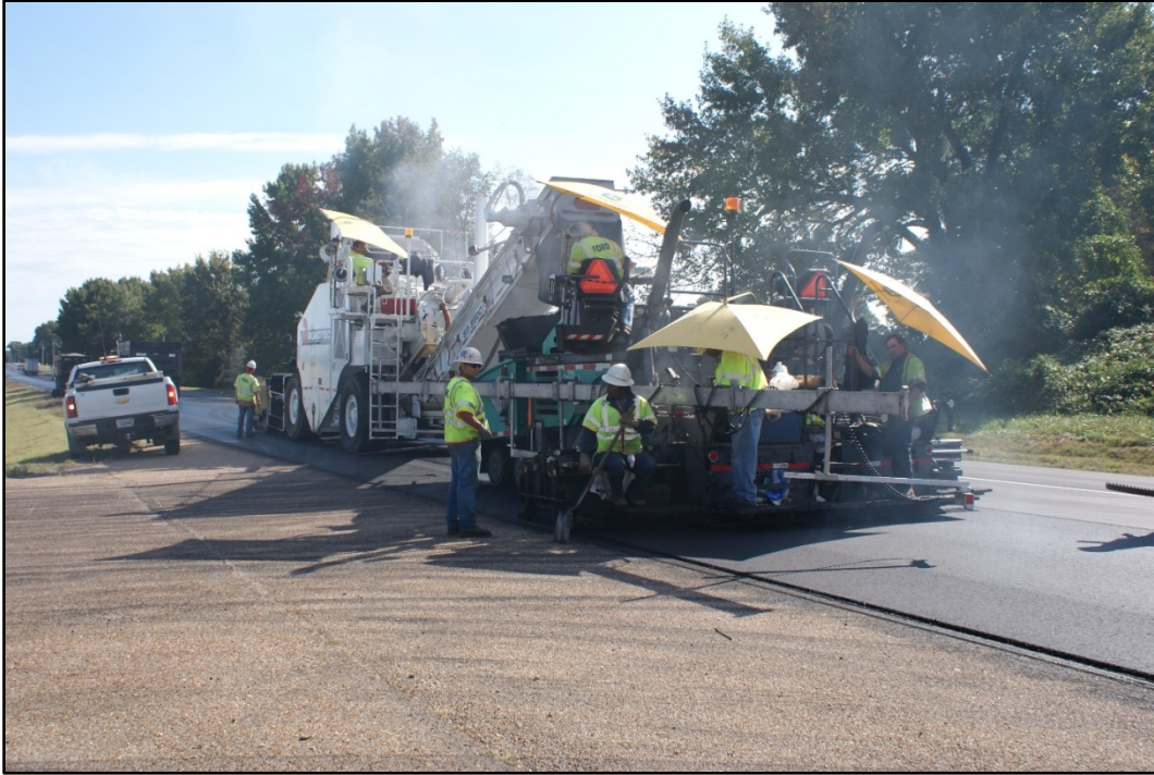
Figure 21. Photo. Typical AC placement.
