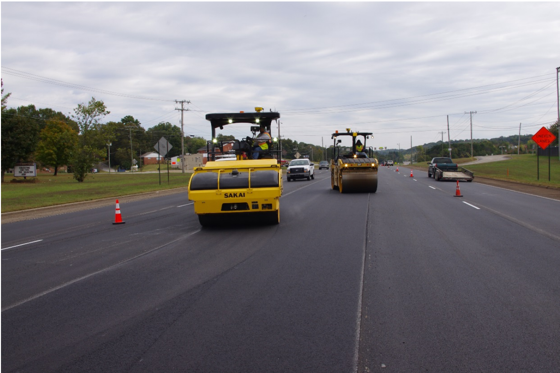
Figure 30. Photo. IC roller in operation. (courtesy: TDOT)
