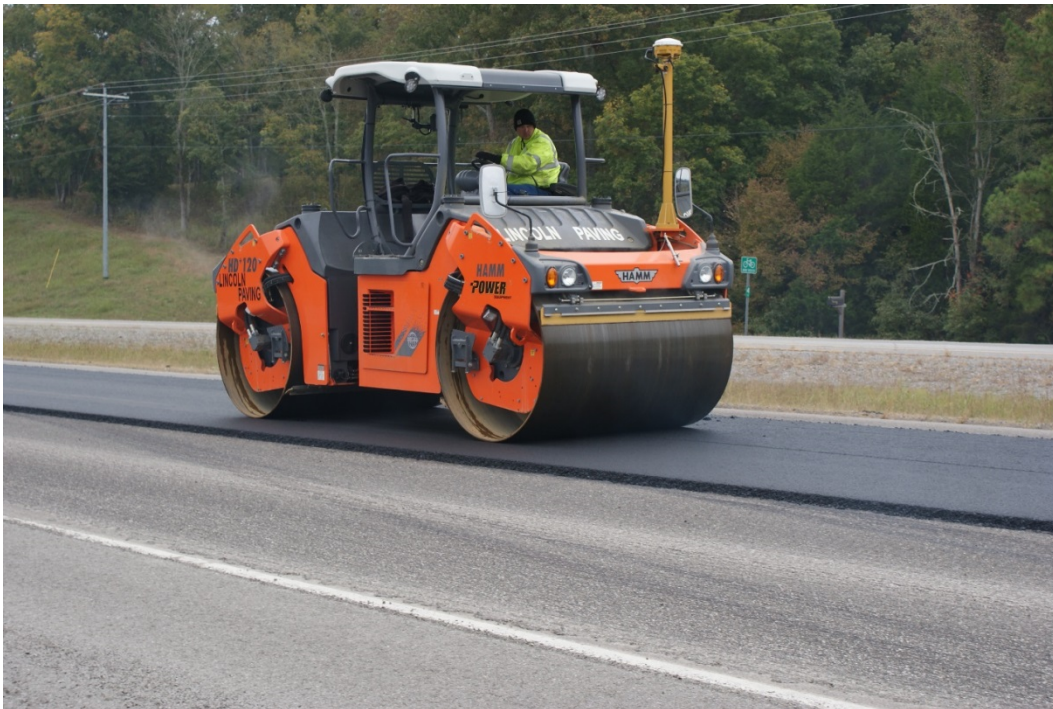
Figure 38. Photo. IC roller in operation.
