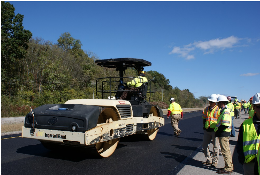
Figure 42. Photo. Observation of IC roller on AC surface course.
