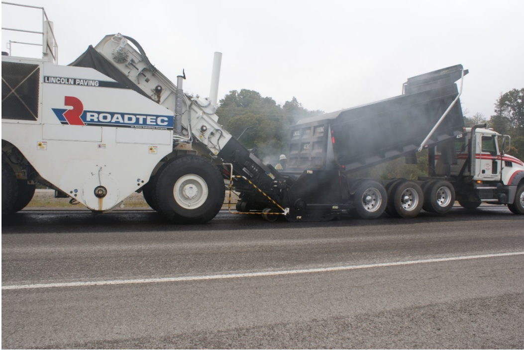
Figure 37. Photo. AC mat placement.
